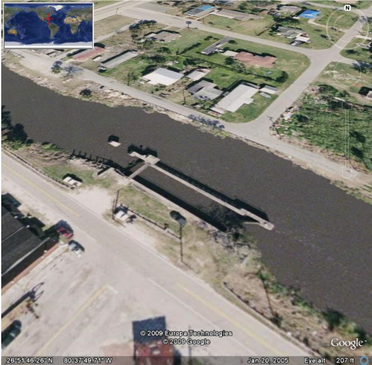
Google Earth view of Canal Point Lock Canal Point, FL southeast of Lake Okeechobee
