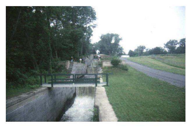
Glens Falls Feeder 5 Combined locks, # 6 -10 7/9/94 Locks being used as flume
