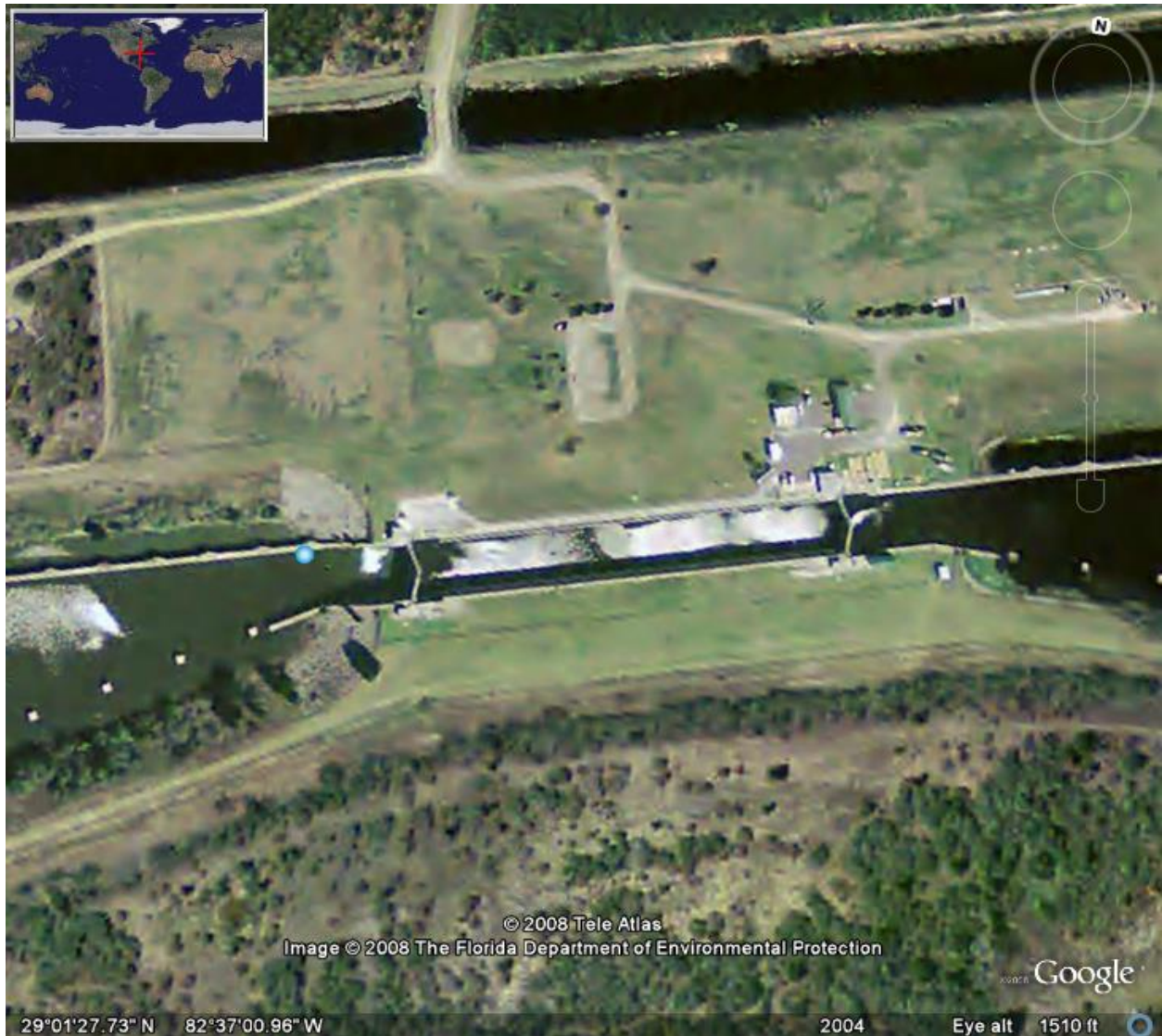
Google Earth view of Inglis Lock Cross Florida Barge Canal
