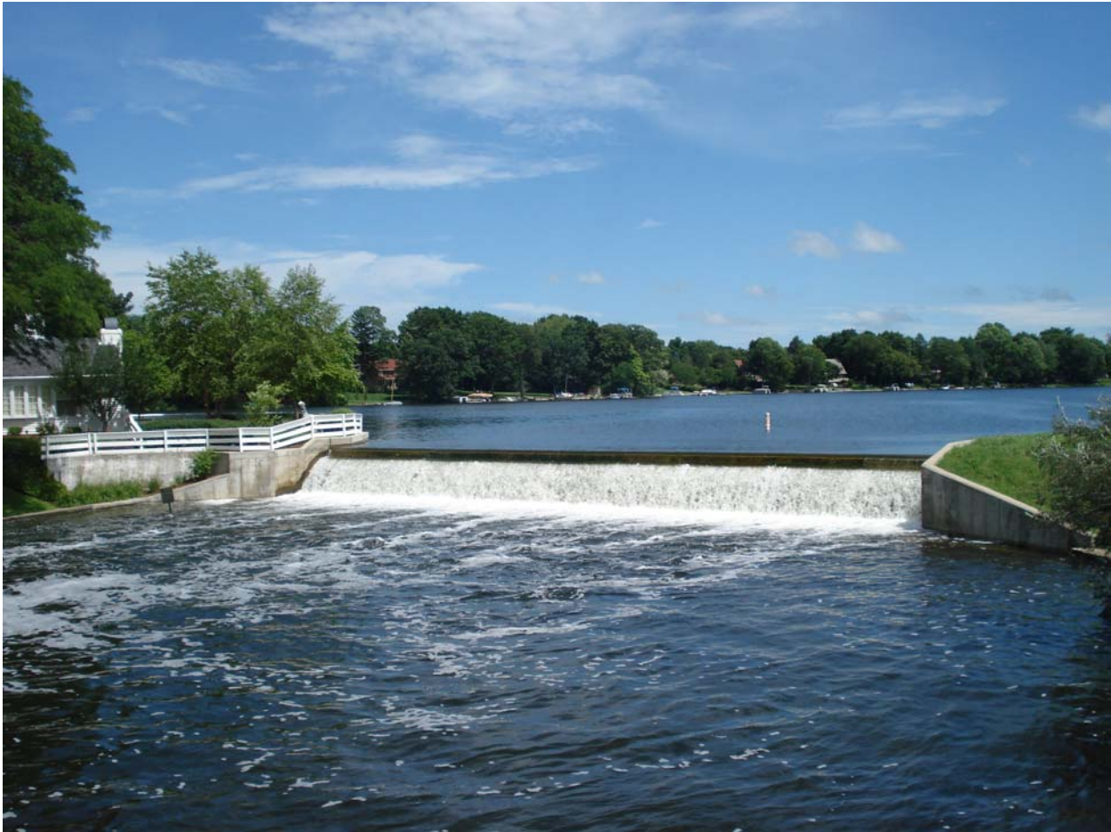
The dam from Fowler Lake to Lac La Belle at Oconomowoc, WI Most likely, the lock was to the left of the dam in this photo where a house now sits.
