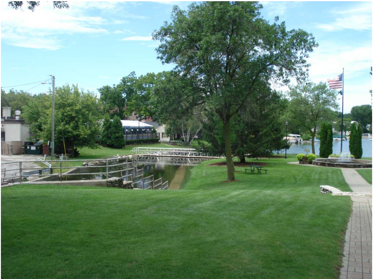
View in the opposite direction of approximate route of boat railway, Oconomowoc, WI
