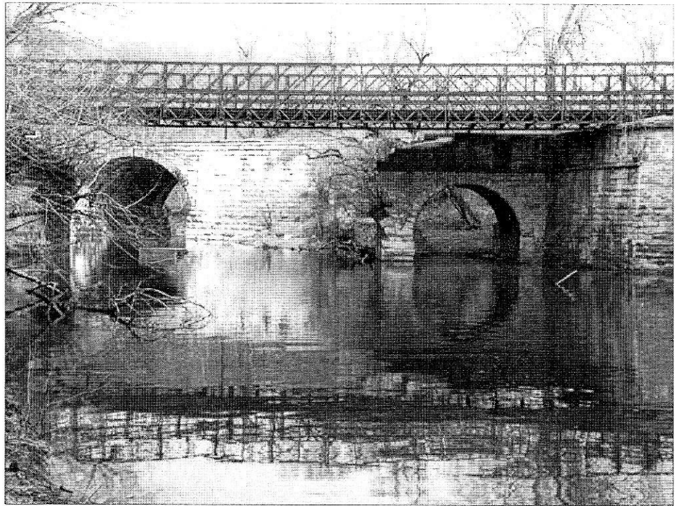
This picture is a combination of three elements: the single remaining arch of the Catoctin Creek Aqueduct, on the right (the missing two arches collapsed in 1973); behind it an arch of the B&O railroad bridge; and on top of them both is the steel and wood foot bridge NPS built after the collapse. http://canal.mcmullans.org/participate.htm .
