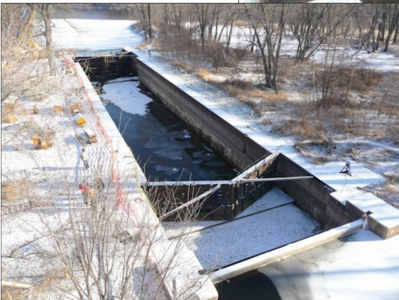
The rebuilt lock with the stop logs still in place 12/24/11 photo by Ed Kirchhoff
