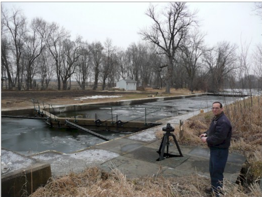
The rebuilt lock with the stop logs removed and Berlin Boat Club commodore Ed Kirchoff 12/30/11 photo by Dick Schramer
