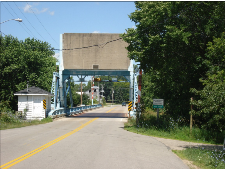
Eureka lift bridge 7/11/09 photo by Dave Barber
