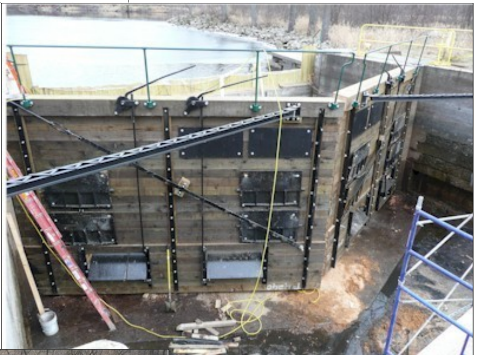
The rebuilt lower gates 12/20/11 photo by Ed Kirchhoff
