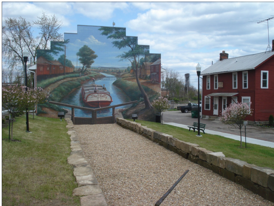
Ohio & Erie Canal, Lock 9 north, Newark, OH, 4/12/12 showing the restored lock, mural, and lock house. Photo by David Barber.
