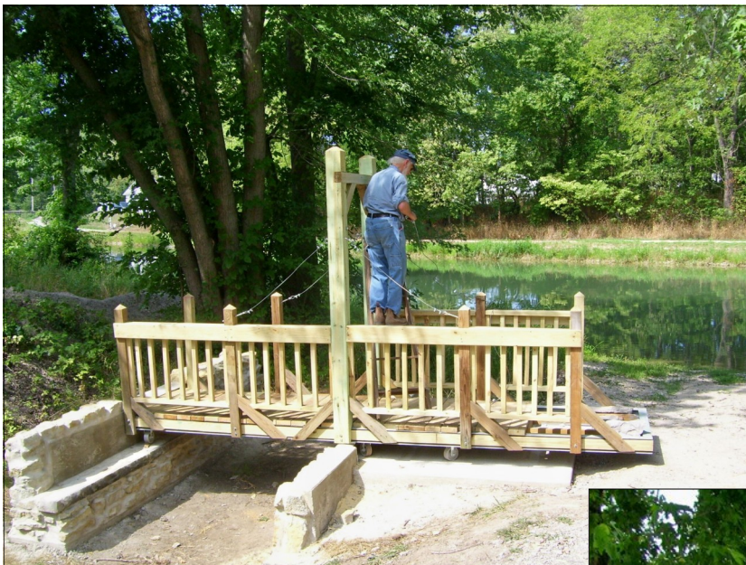
Roy working on the cabling for the bridge. ▼
