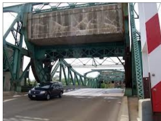
Jefferson Street Bridge, Joliet, Illinois
