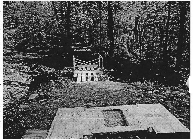
View across the abutments and staging before bridge installation
