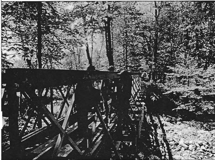
Volunteers completing fiberglass construction ▼
