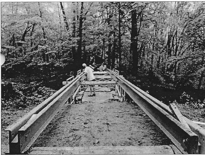
▲ Lower bridge channels installed
