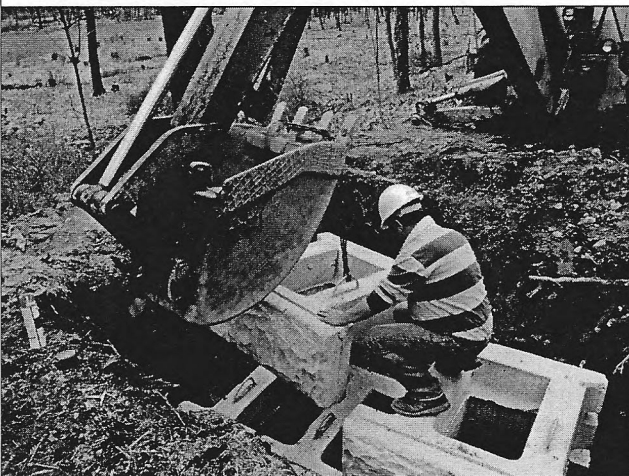
Abutment being assembled
