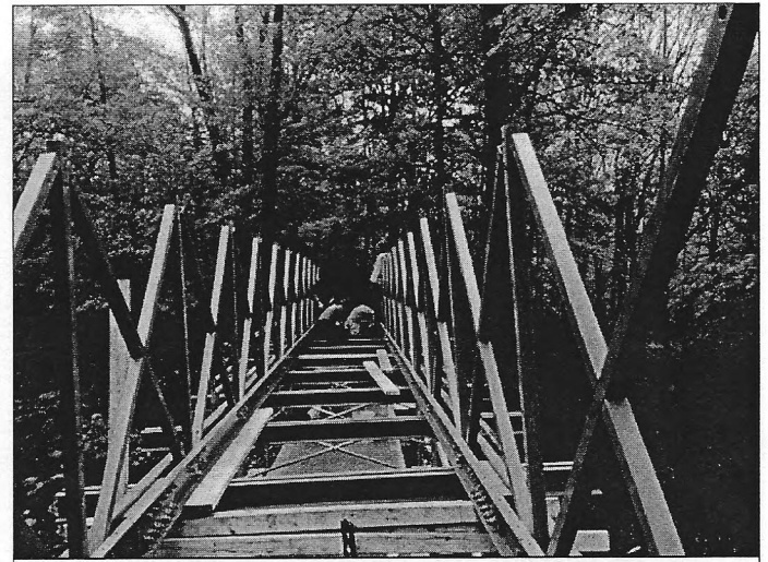
▲ Cross bracing and cross channels installed
