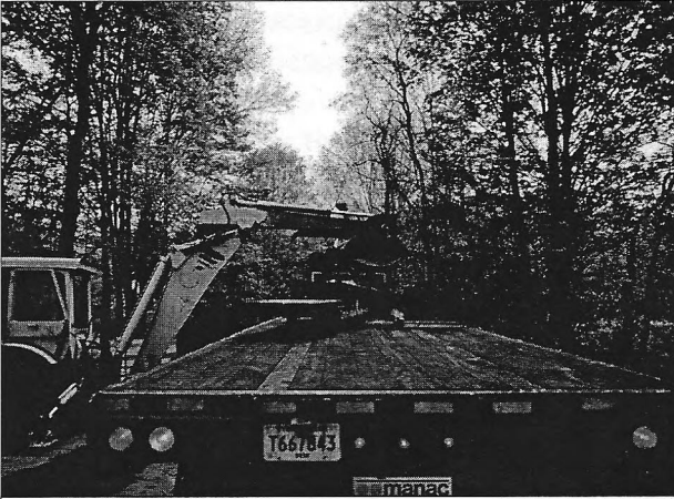
Unloading bridge members
