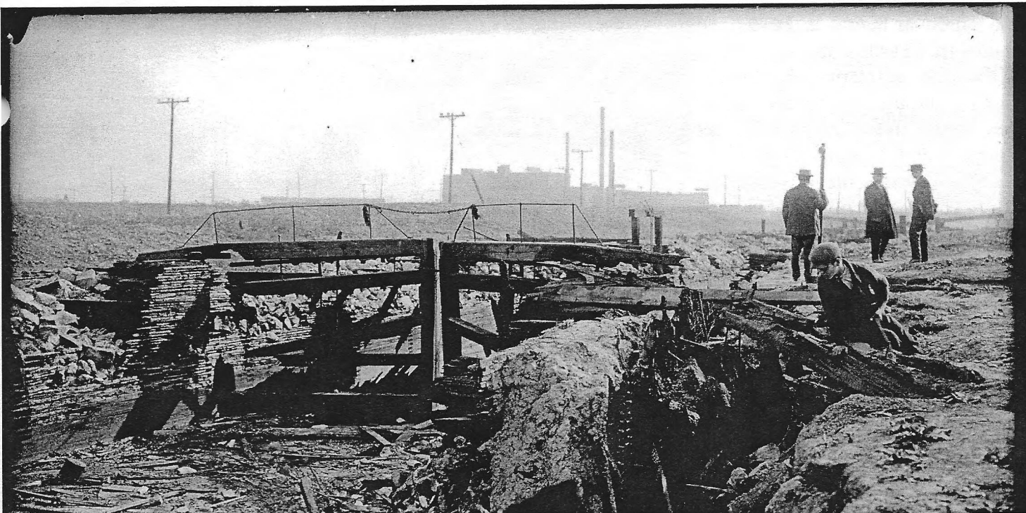
Bridgeport Lock looking south, Note that this is a wood crib lock. 5/2/14
