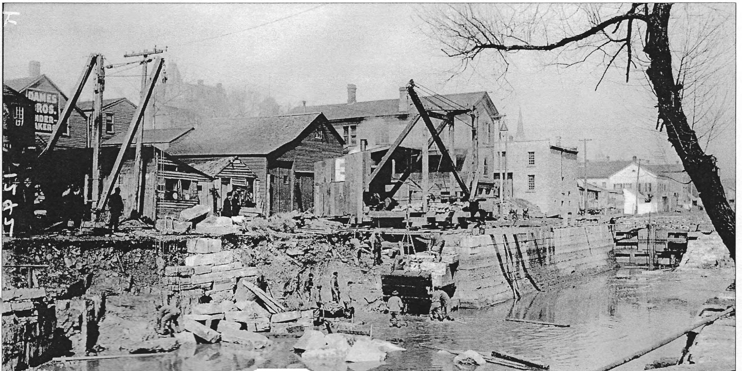
Dismantling of Joliet Guard Lock, March 1899
