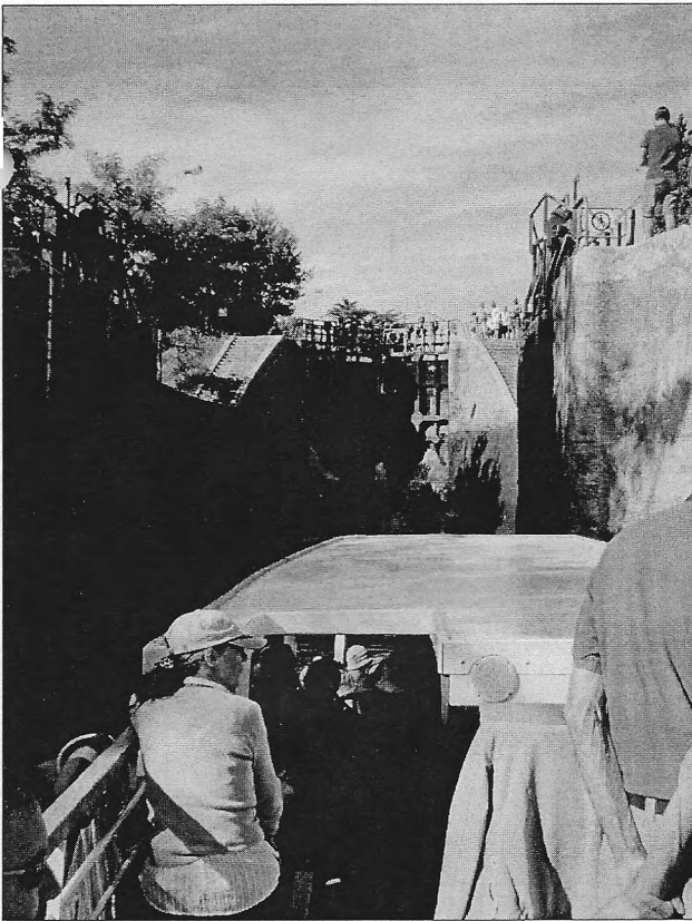
The Fonserenes staircase of locks consists of eight curved lock chambers (characteristic of the Canal du Midi) and nine gates that allow boats to be raised a height of 21.5 meters in a distance of 300 meters.
