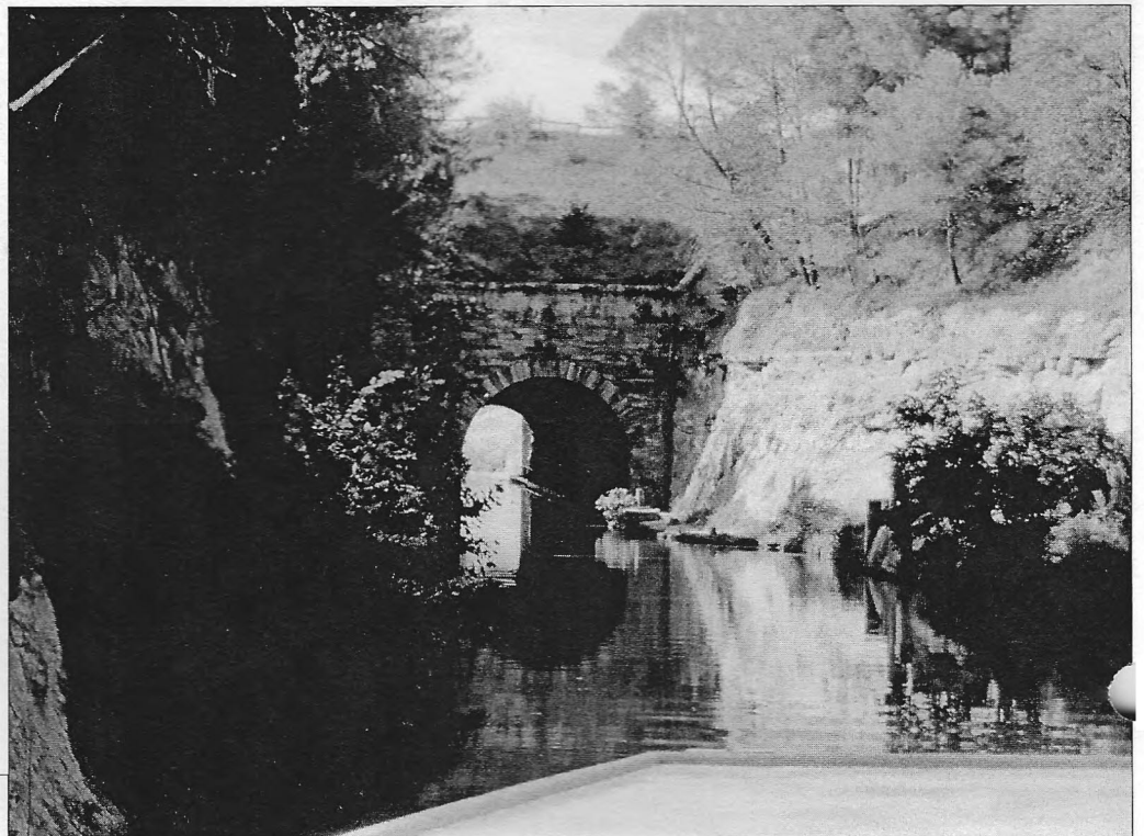
The exterior of the Malpas tunnel.
