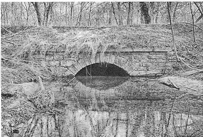
C&O Canal Culvert 91 towpath arch. Photo by Steve Dean
