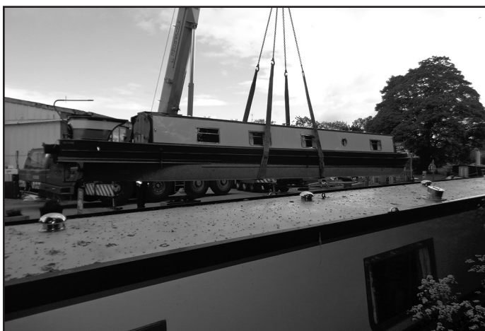
Craning a narrowboat into the canal at Hanbury Wharf
