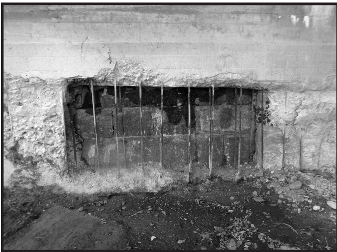
A test area on the viaduct where the concrete was removed to expose the original granite. Photo by David Barber
