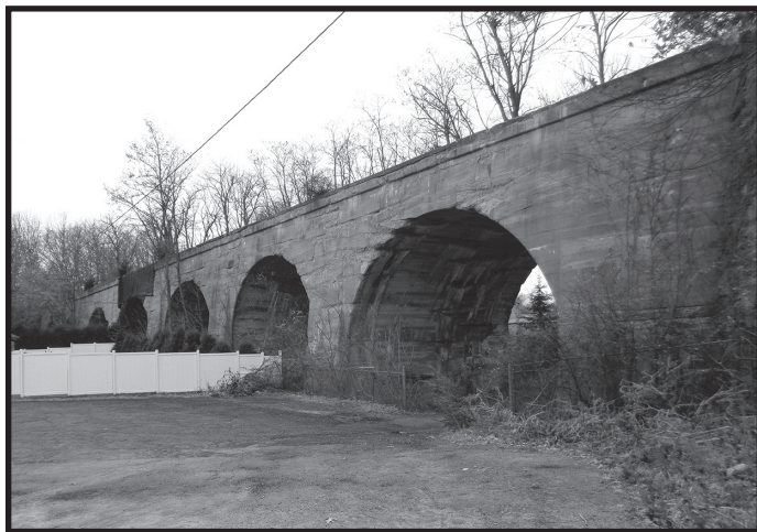
The Blackstone Viaduct. Photo by David Barber
