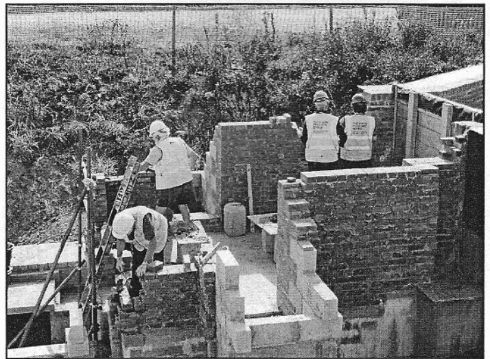
Figures 5 (above) and 6 (below): Chesterfield Canal Trust work party and Waterway Recovery Group work party constructing the Staveley Town lock. Figure 6 courtesy Chesterfield Canal Trust.
