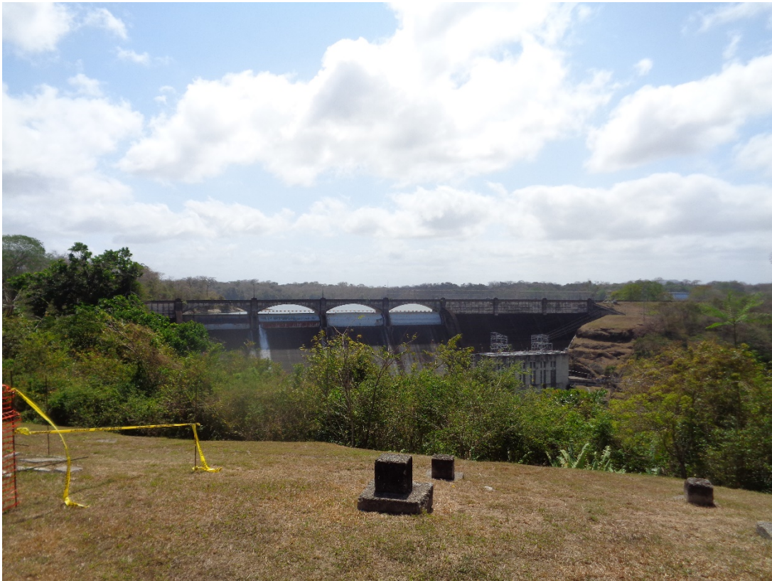
Madden Dam on the Chagres River 3/6/17. This dam creates a reservoir to store water for canal operations.
