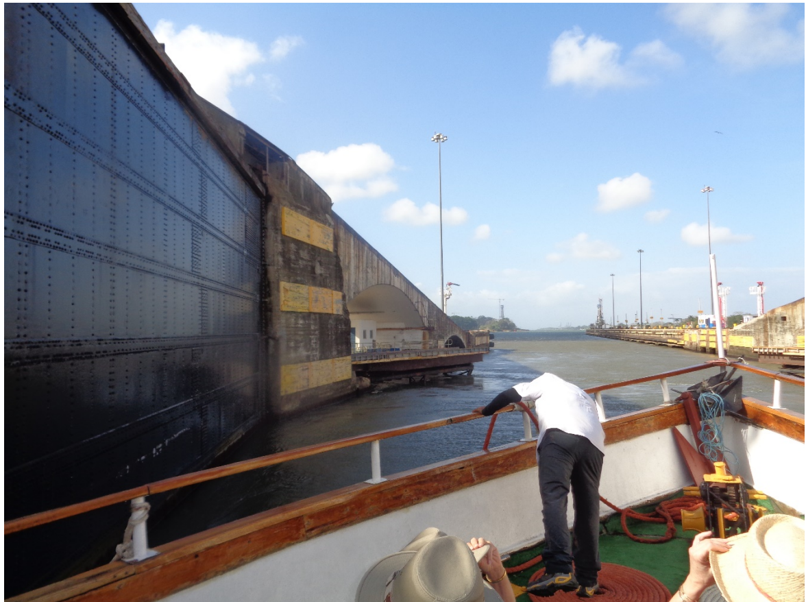
Looking north from exit of Gatun Locks 3/7/17. Roadway bridge at north end is opening.
