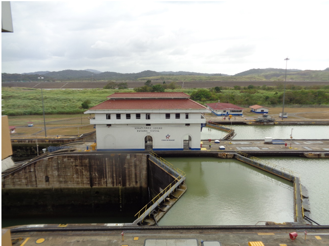
The control house at Miraflores Locks viewed from the visitors center 3/6/17
