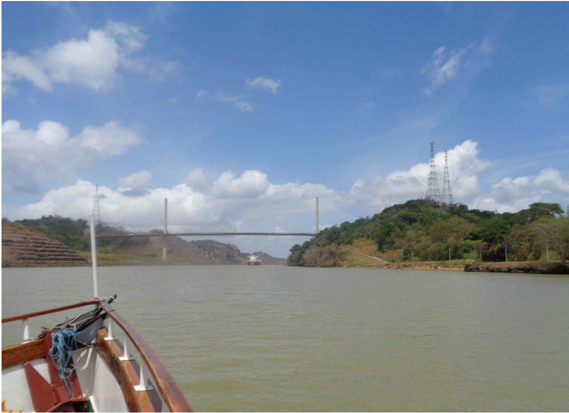
Approaching Culebra Cut and the Centennial Bridge northbound 3/7/17
