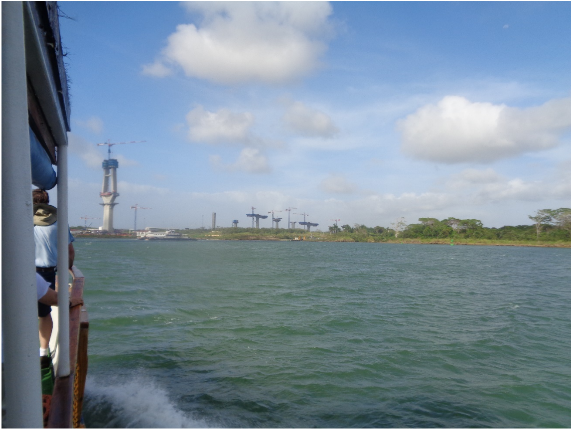
New bridge under construction 3/7/17 north of Gatun Locks.
