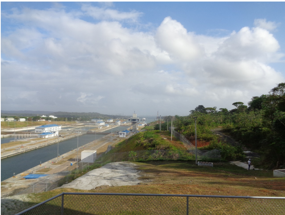
View of the new Atlantic end locks looking north from the visitors' center on 3/8/17. Looking diagonally across the near lock, a white cruise ship is visible above the blue-roofed buildings waiting to enter the older locks.
