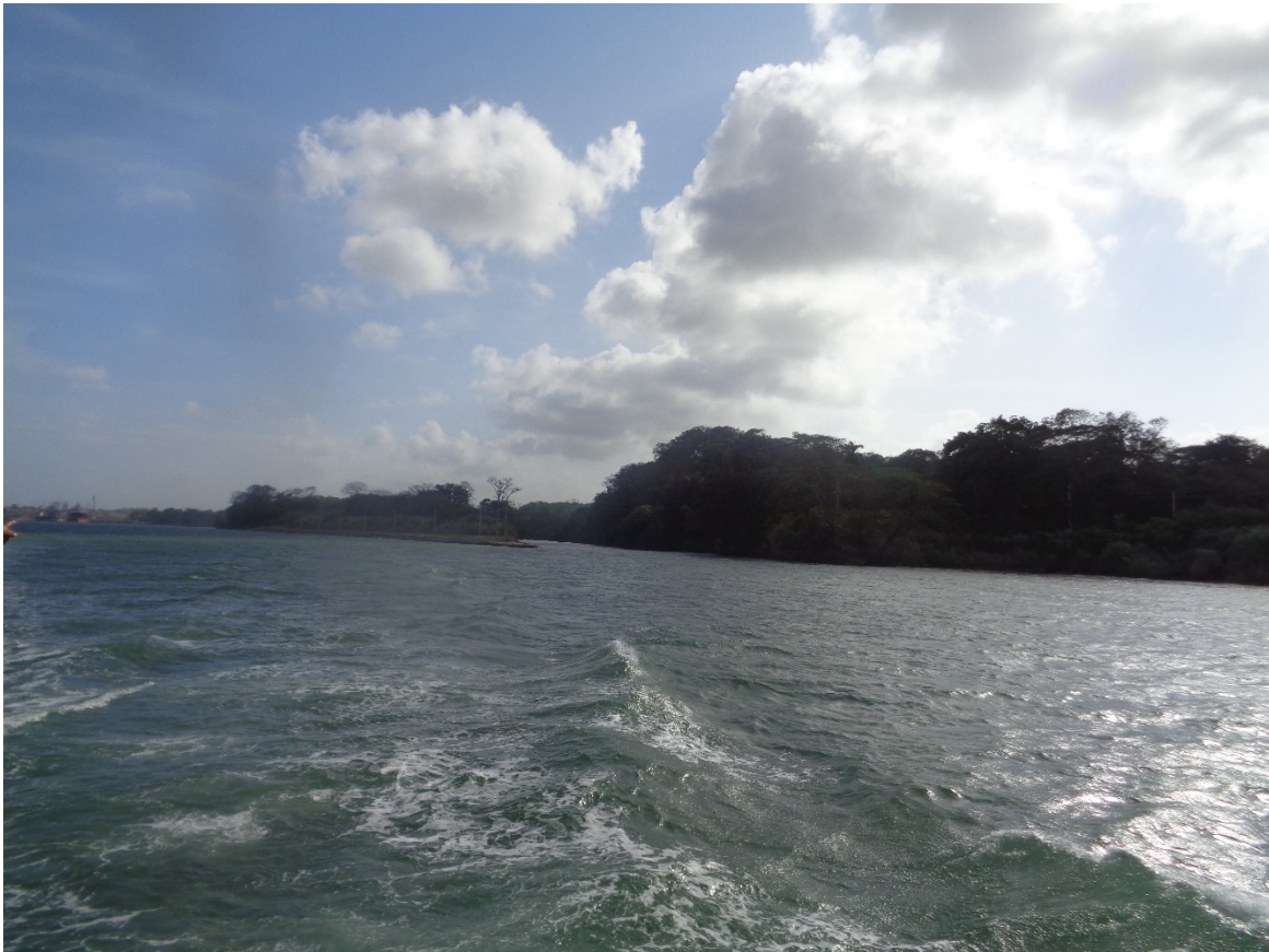
Junction of canal with French Canal north of Gatun Locks 3/7/17. French Canal is to right.
