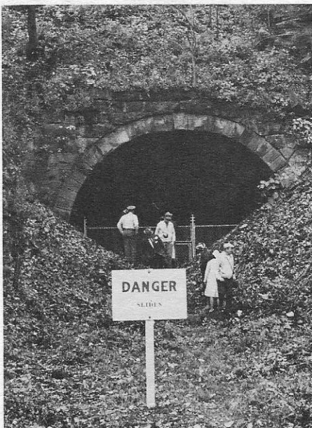
One of the portals of the Main Line Canal Tunnel as it looked about 1970. (Photo by Bill Shank)
