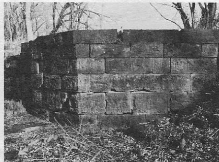
The east wall of the sidecut's lower gate-support structure.
