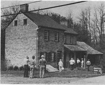
Restored Lockhouse, just south of the flight of Locks, Numbers 52 and 53, at Leesport.
