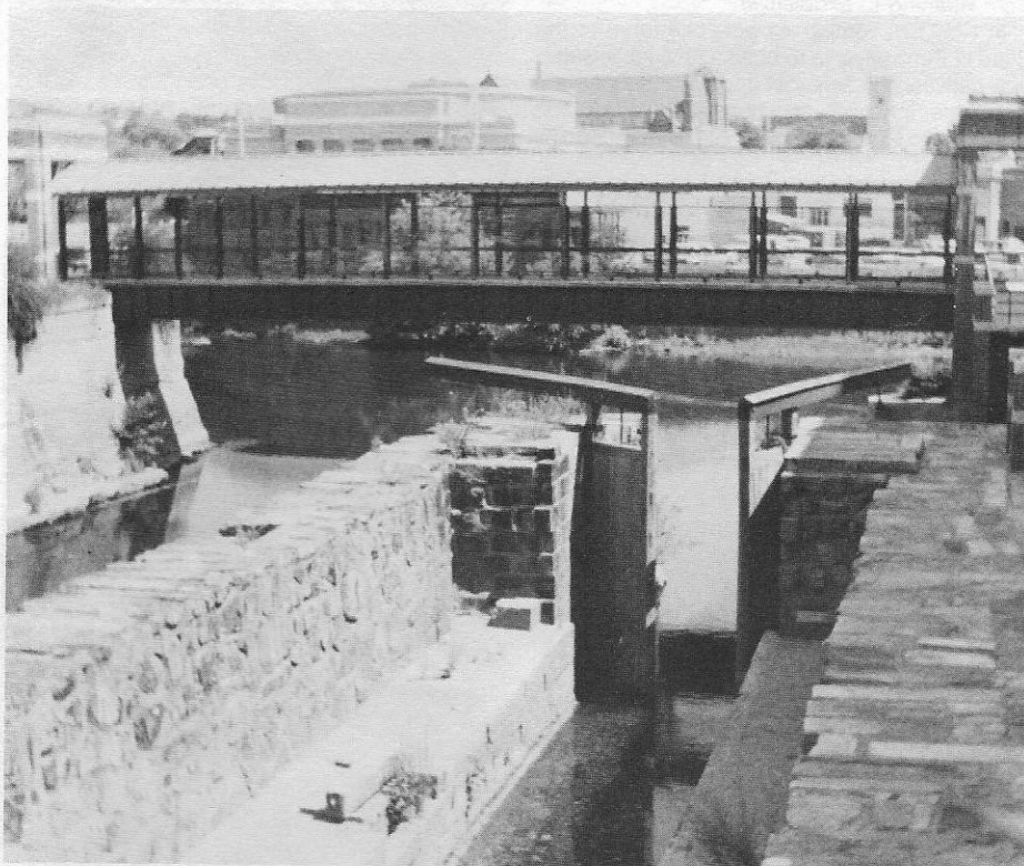
Restored lock chamber and gates in Lowell.
