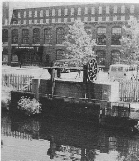
Mechanism for controlling flow of water on one of Lowell's canals.
