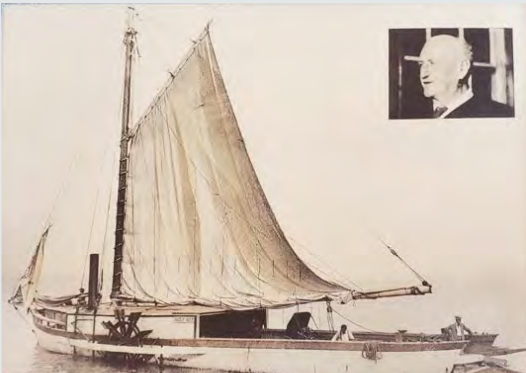
The Busy Bee , a Cayuga Lake Ferry. The Busy Bee was built for service between Kings Ferry and Kidders. She was 67 feet overall length with a beam of 17 feet, and could be powered by sail or steam. At the height of her activity she made regular trips every day to meet the trains and carry mail and was steered by a rudder that was a heavy detachable paddle. The ferry was owned and operated by Captain James Quick (inset), who operated ferries until trains and automobile put him out of business. Research indicates the Busy Bee was abandoned and we expect to locate it when the survey extends into Cayuga Lake.
