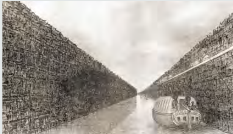
Building the Erie & Champlain Canals was a triumph of engineering. The deep cut west of Lockport allowed Lake Erie water to supply the western end of the canal from Buffalo to the Seneca River. The flight of five locks at Lockport (bottom) were a great engineering feat. From Cadwallader D. Colden, Memoir prepared at the Request of the Committee of the Common Council of the City of New York , 1825. Canal Society of New York State
