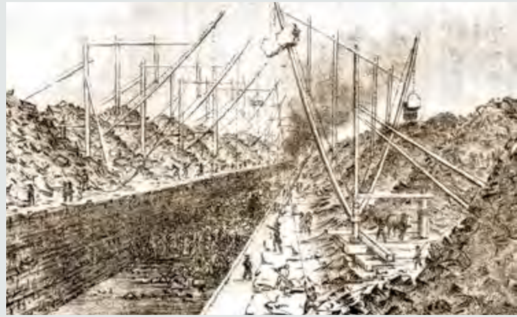
Building the Erie & Champlain Canals was a triumph of engineering. The deep cut west of Lockport allowed Lake Erie water to supply the western end of the canal from Buffalo to the Seneca River. The flight of five locks at Lockport (bottom) were a great engineering feat. From Cadwallader D. Colden, Memoir prepared at the Request of the Committee of the Common Council of the City of New York , 1825. Canal Society of New York State
