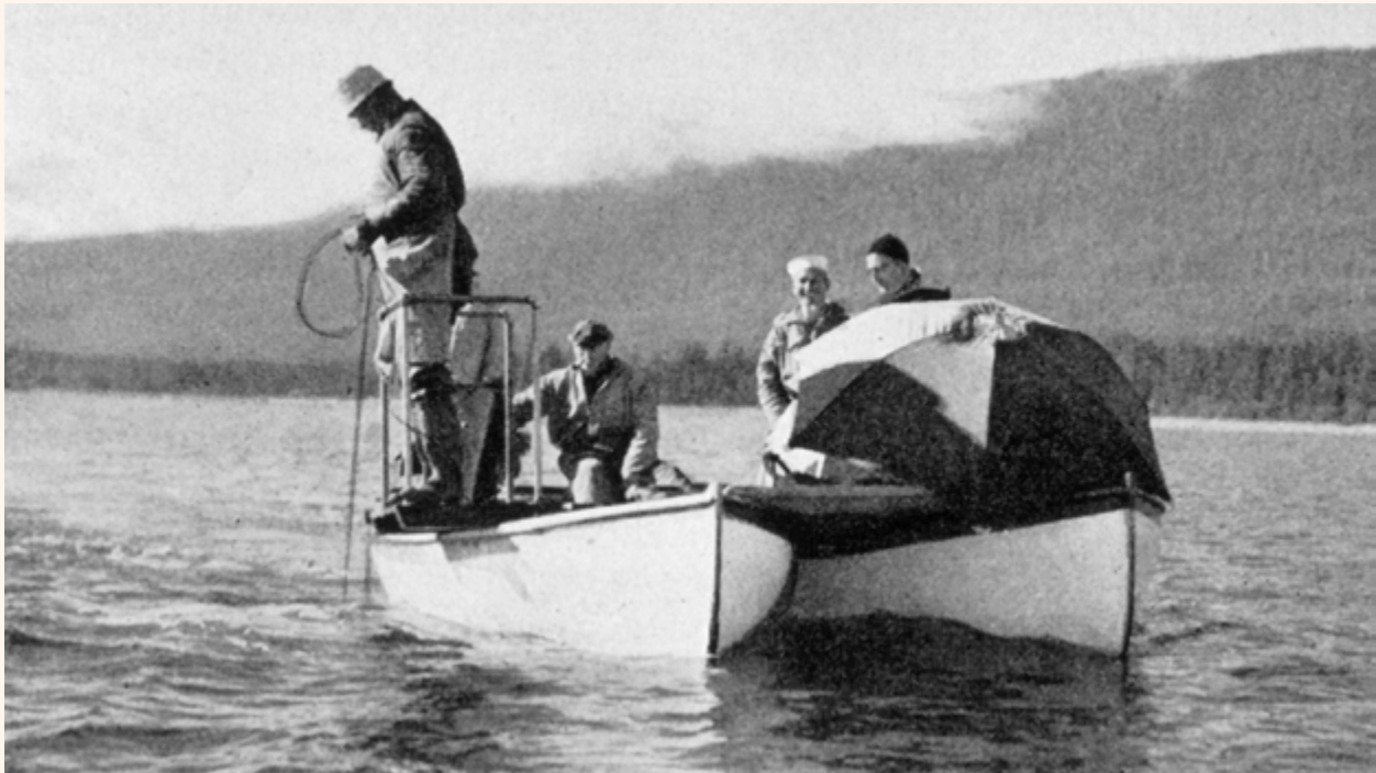
Figure 1: Example of a lead-line observation in a lake. National Oceanographic and Atmospheric Administration
