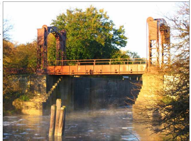
Wyanet lift bridge over the Hennepin Canal
