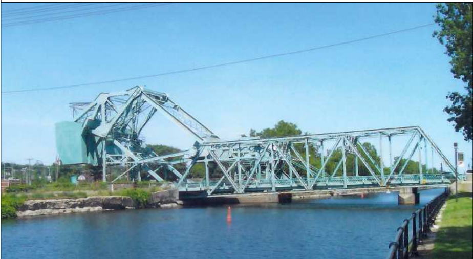
A bascule bridge spanning the Lachine Canal dates from the early 20th century, a time when the waterway was in constant use by vessels up to 265 feet long.
