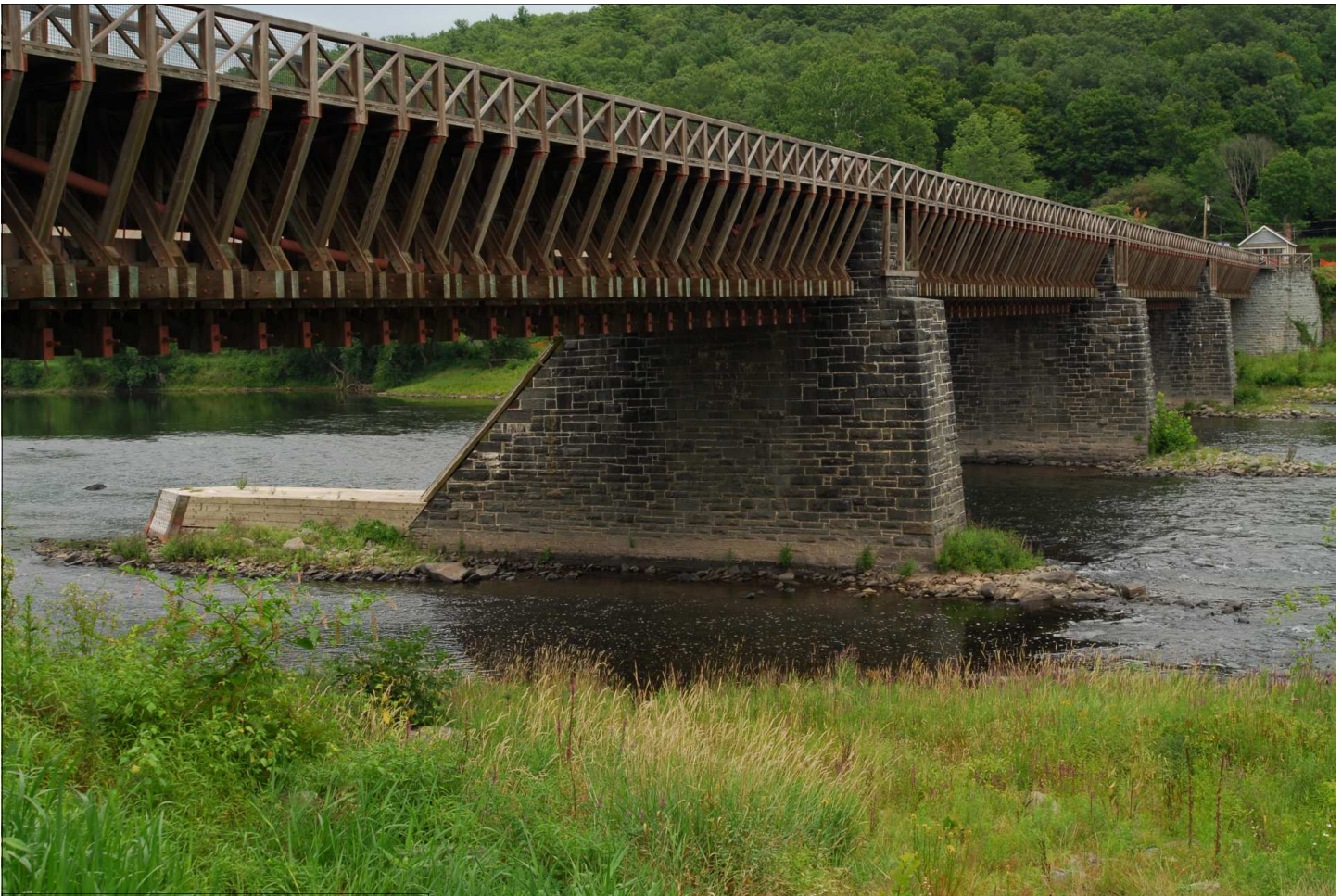
The Delaware Aqueduct carried the D&H Canal across the Delaware River.
