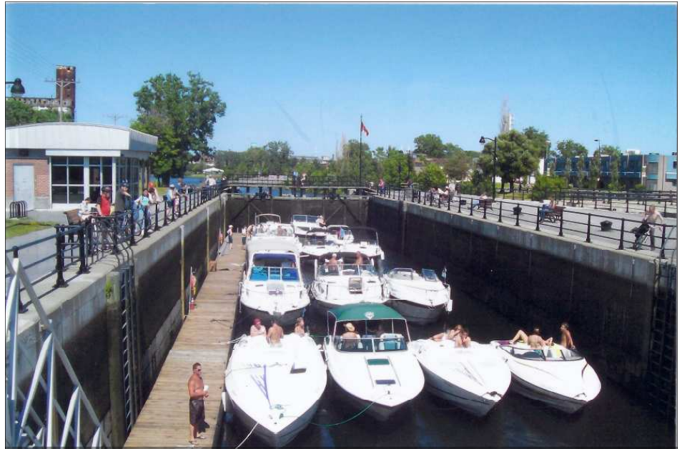
The locks of the Lachine Canal are now used only for pleasure craft. During the busy summer boating season, it's customary to wait until there are enough boats to completely or partially fill the lock chamber. Boats using this canal overcome about 50 feet as they bypass the treacherous Lachine Rapids.
