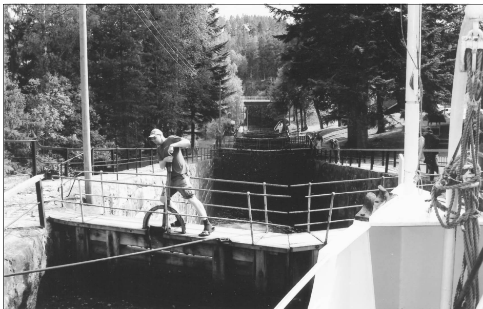
Lockkeeper lifting a paddle at the top of the Vrangfoss flight, Telemark Canal Photo by Dave Johnson
