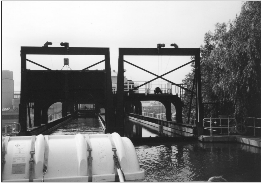
A view from the top of the Anderton lift, showing the caissons filled with water. The caissons move vessels between the River Weaver and the Trent & Mersey Canal.
