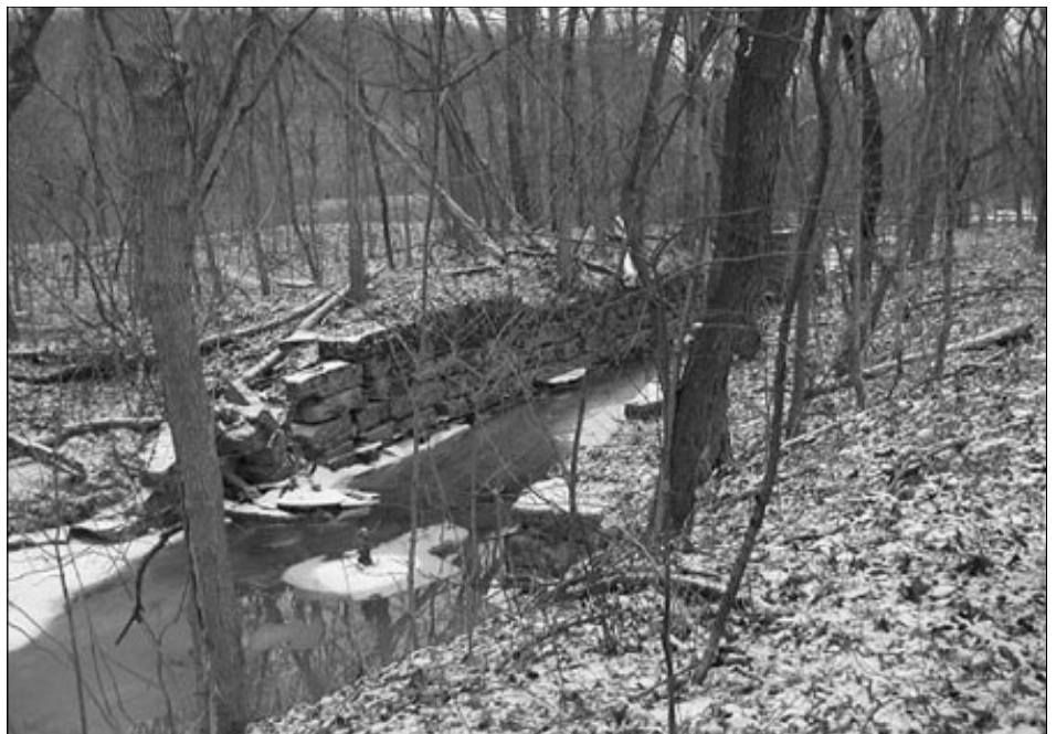
Lock 23 on the Whitewater Canal at Twin Locks south of Metamora, will be the northern starting point for the newly funded Whitewater Canal Trail segment. Photo by Mick Wilz.
