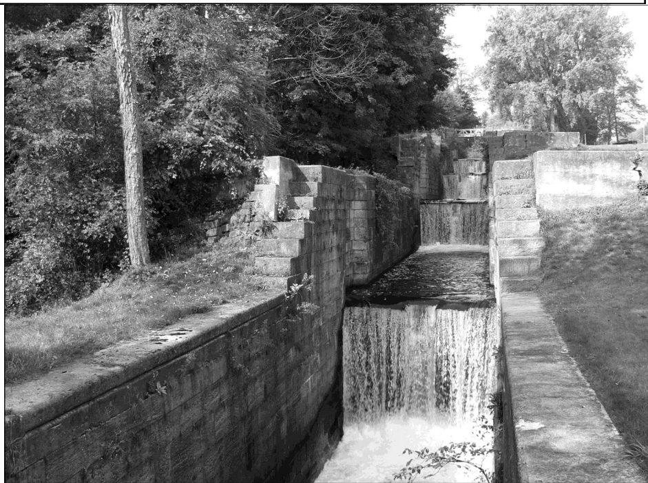
The five-lock combine on the Glens Falls Feeder Canal. The water is feeding the Champlain Canal, as it has done since 1823. Photo by Jakob Franke. See story on page five.
