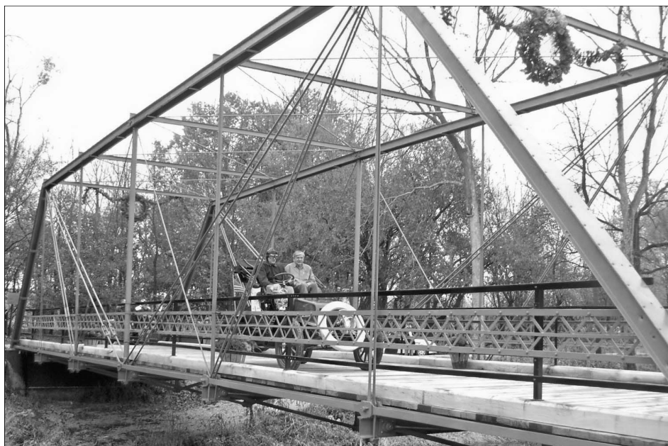
1903 Winton automobile crossing the Wabash & Erie Canal on the 1905 wrought iron Stearns truss bridge. Photo by Dan McCain.
