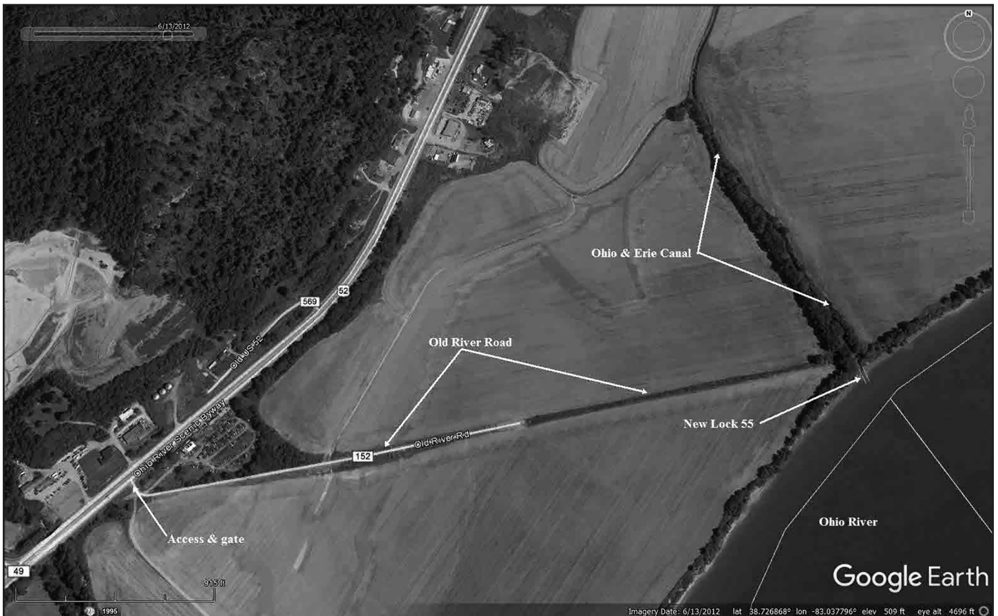
Aerial view of New Lock 55 and the access road - Image courtesy of Google Earth
