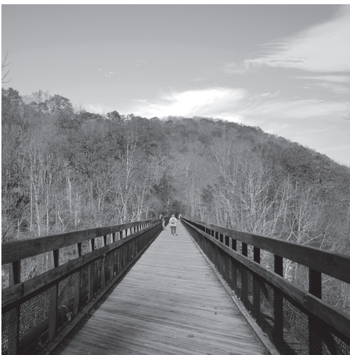
Top – Potomac River near Antietam Creek Center – Fifteen Mile Creek Aqueduct Bottom – Great Allegheny Passage bridge over the Youghiogheny River
