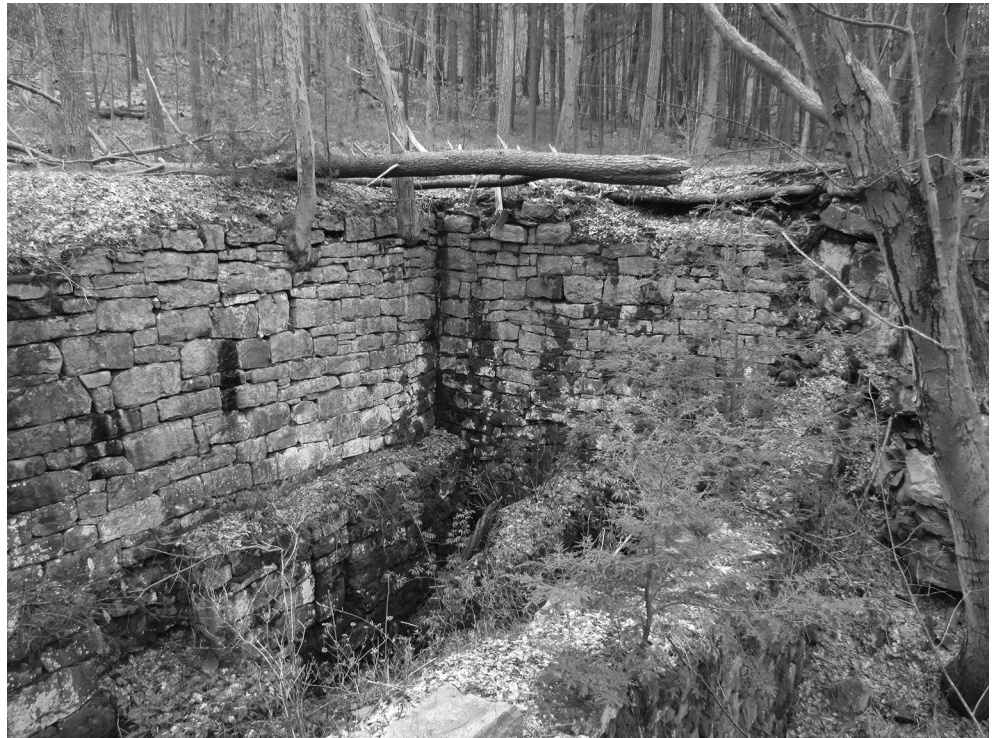
This is stonework in the engine house at the top of old Plane 2. The recess at the bottom was likely for 20 foot diameter wooden winding wheels. The depth suggests the tracks at the top of the plane went over the top of the engine house, similar to the Switchback Railroad planes at Jim Thorpe. Later engine houses were three stories and the tracks at the top curved to one side of the house. The two story height of the operator provided a clear view of the plane. Later winding wheels were made of steel and built by Bethlehem Steel. Photo by Doug Logan
