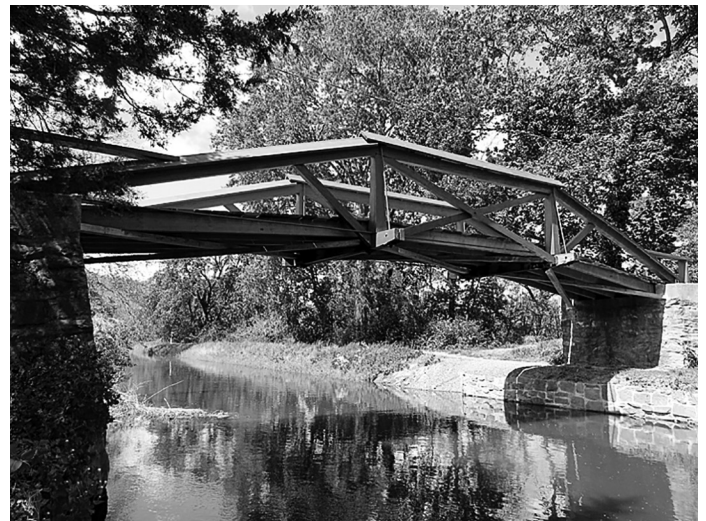
Woody's Camelback Bridge in its finished glory. Photo by Carole Mebus
