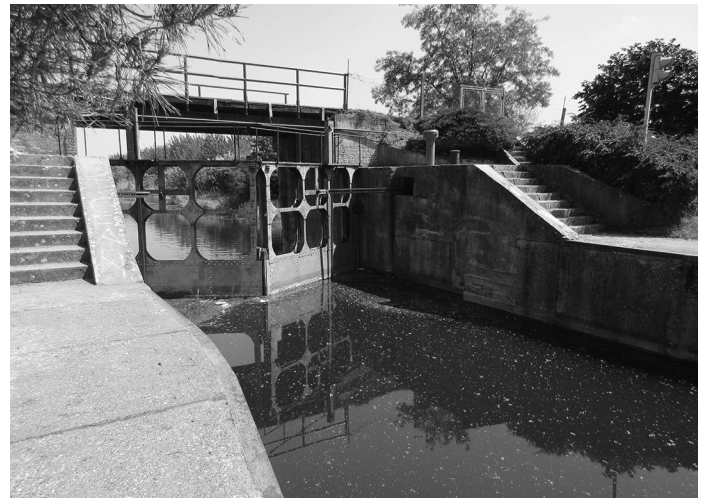
Mali Stapar lock on the Bezdán-Vrbas Canal – Photo by Chris Holdsworth
