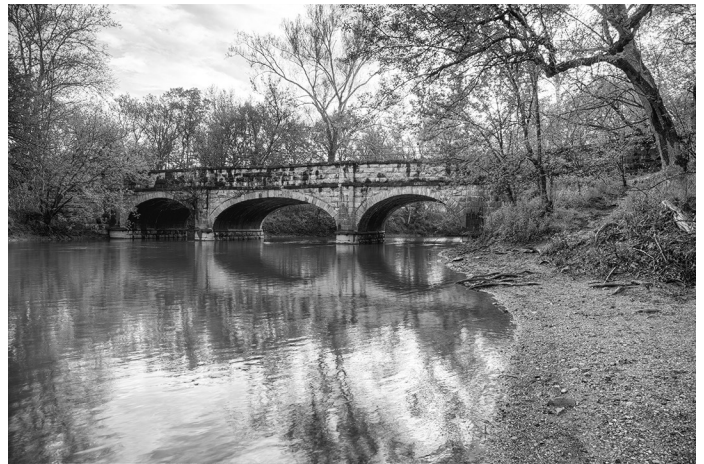
Antietam Creek (mile 69.36) – Featuring elliptical arches, this aqueduct survived Civil War damage. The center arch is wider than the upstream and downstream arches.
