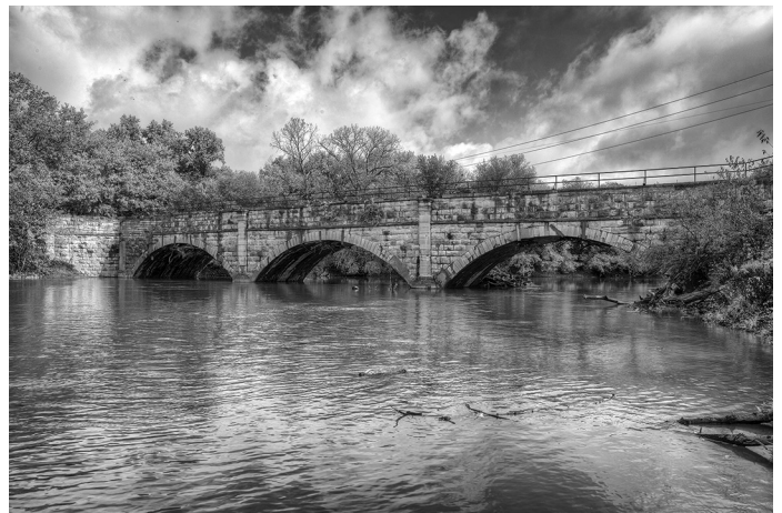
Conococheague Creek (mile 99.80) – A canal boat went through the side of this aqueduct in 1920. A restoration project is in progress and eventually boats will again cross it.
