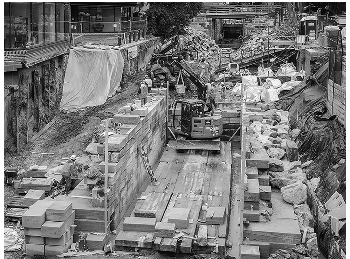
View of Lock 3 toward Thomas Jefferson Street – Photos by Nancy Benco
