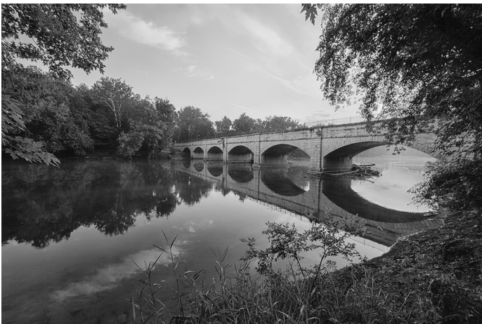
Monocacy River (mile 42.19) – This seven-arch aqueduct is one of the signature features of the C&O Canal. A rehabilitation project, completed in 2005, saved it from possible collapse.
