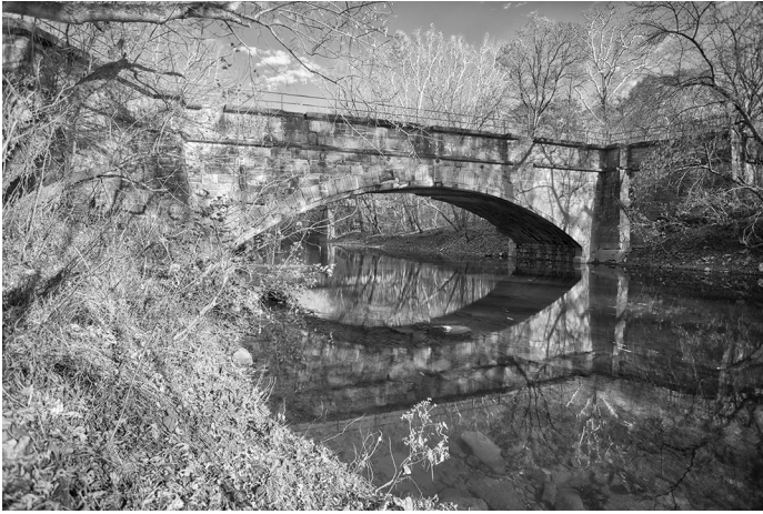
Licking Creek (mile 116.30) – The first of the single-arch aqueducts is also the longest, with a 90-foot span. Weak stones required concrete repairs over the years.
