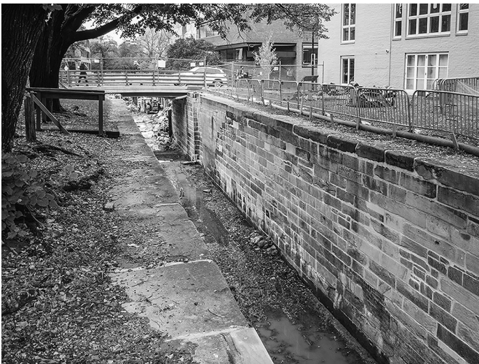
Repointed south wall of Lock 4, view toward Thomas Jefferson Street
