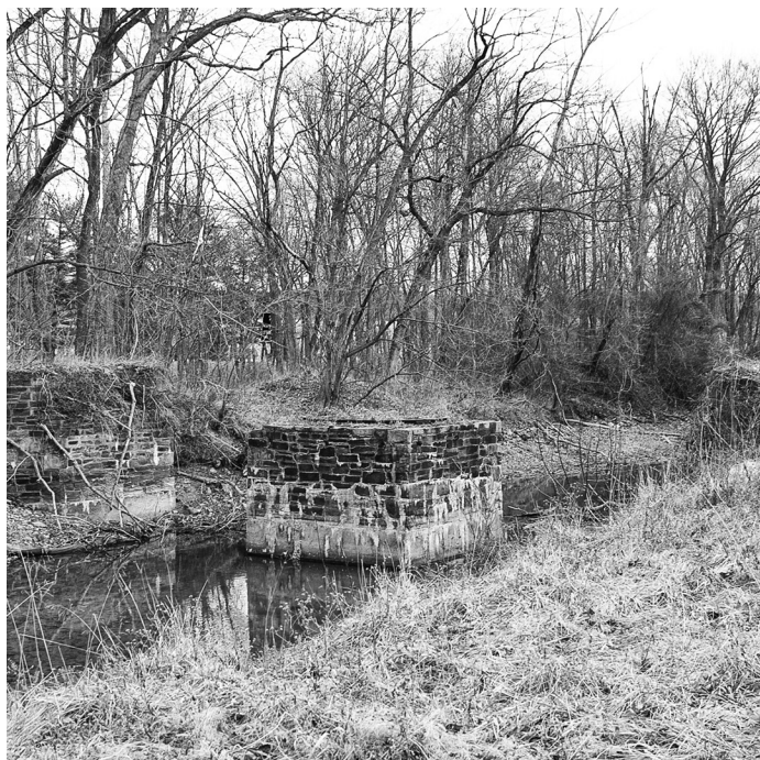
While not a bump bridge, the center pier of a pivot swing bridge is shown in this view from the C&O Canal at Carderock, Md.
