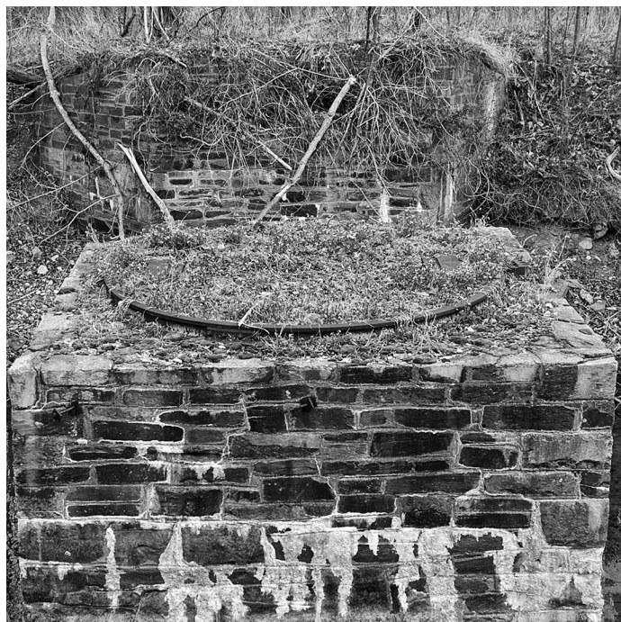
Pivot bridge center pier detail – Photos by Steve Dean
