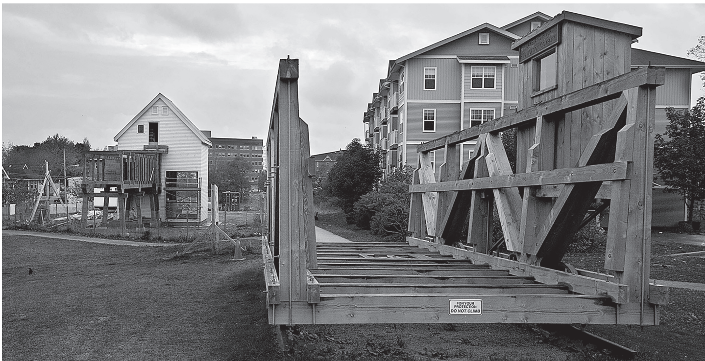
Cradle flume house – Shubenacadie Canal Commission
