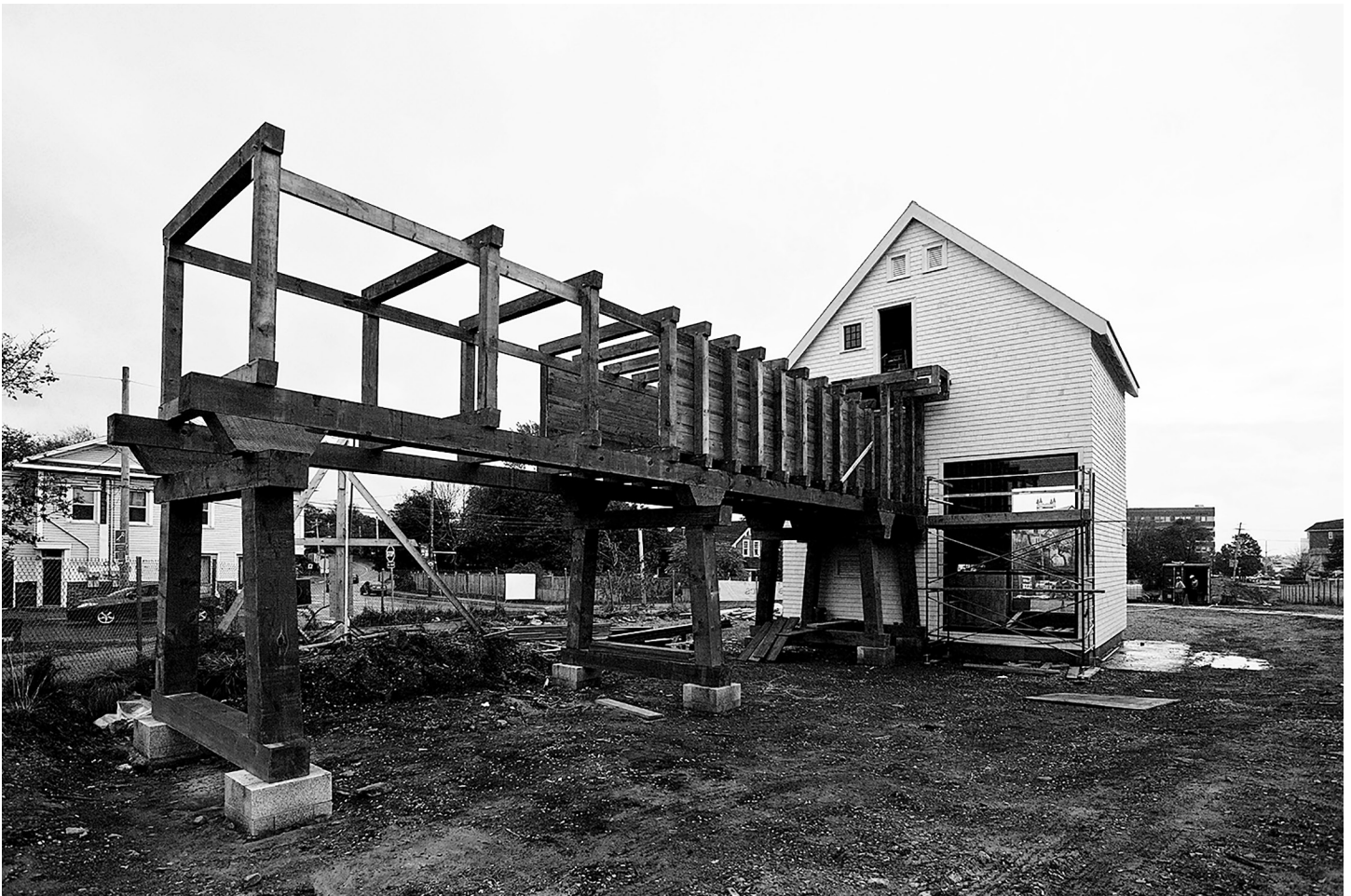
Cradle flume house – Shubenacadie Canal Commission
