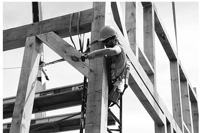
Construction of the flume house – Shubenacadie Canal Commission
