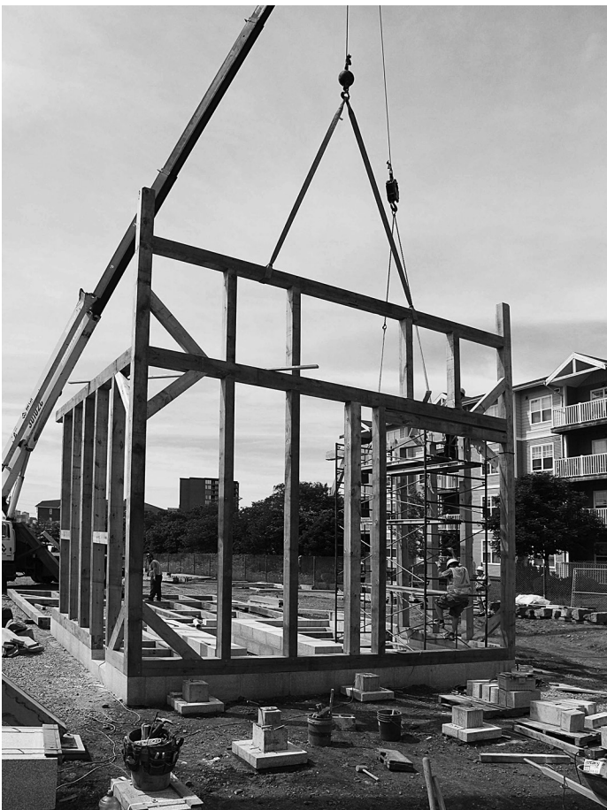
Construction of the cradle flume house – Shubenacadie Canal Commission
