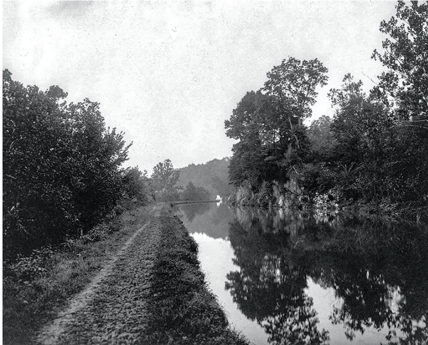
Historic photo of the C&O Canal Towpath at “Log Wall,” miles 10-11 – Courtesy of the National Park Service, C&O Canal National Historical Park
