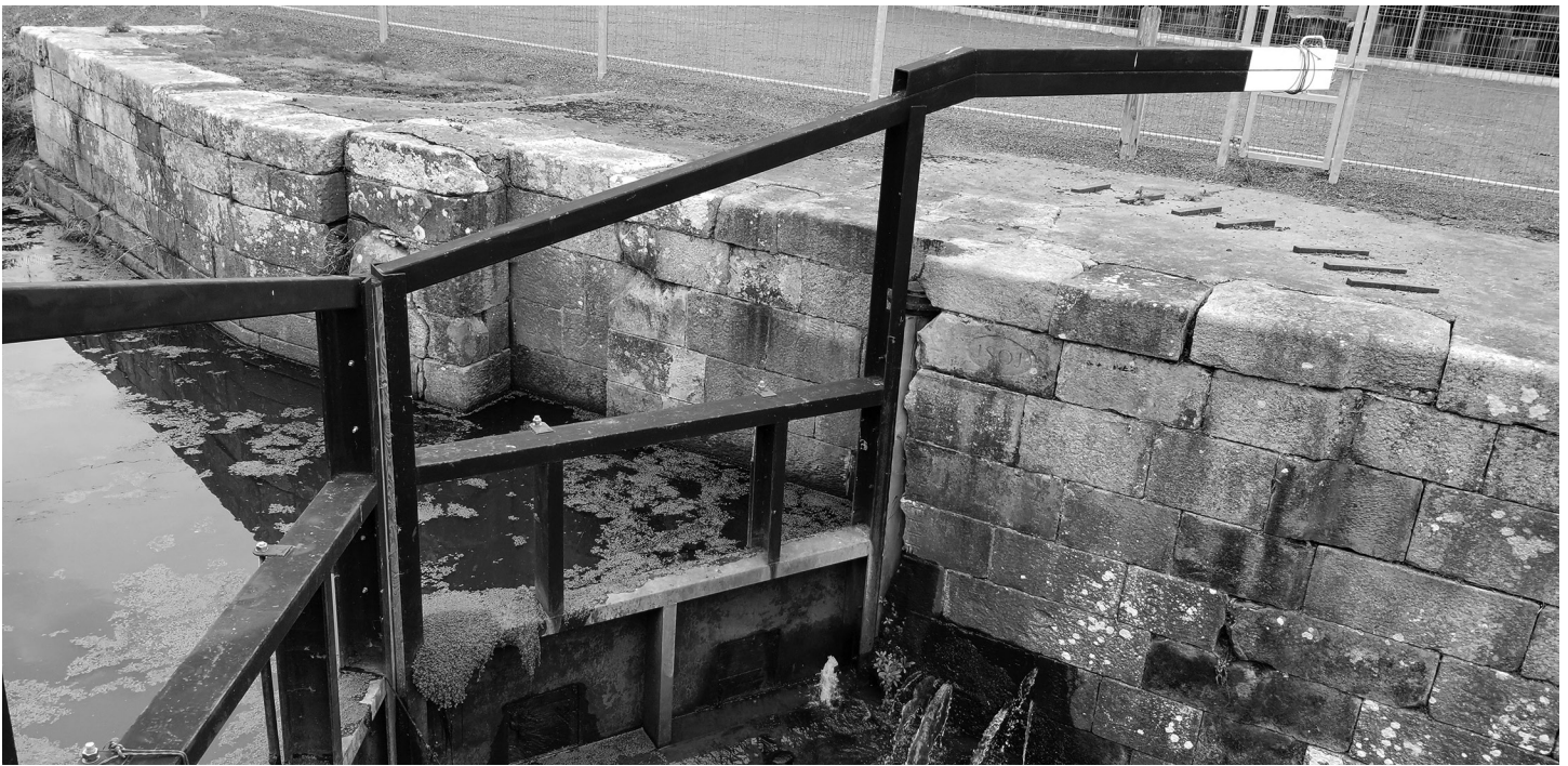
Above – Lock 11 of the Newry Canal, in Poyntzpass. The lock gate was fabricated in 2015 by the local branch of the Inland Waterways Association of Ireland, a voluntary organization. Below – The wayside at Lock 11. – Photos by Rod Mackler
