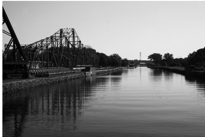
Above – The Canadian Canal with the emergency swing dam
