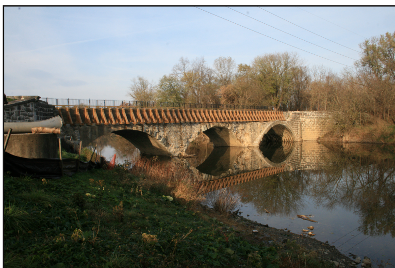
The newly restored Conococheague Aqueduct
