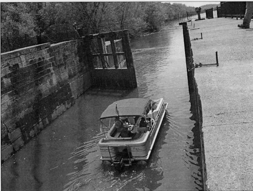
Leaving the Zanesville Tandem Locks. Courtesy, Mark West, Regional Park Manager
