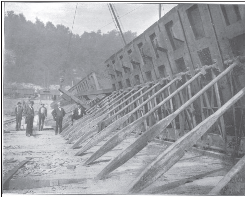
Wicket Gates at Dam 6 on the Ohio
