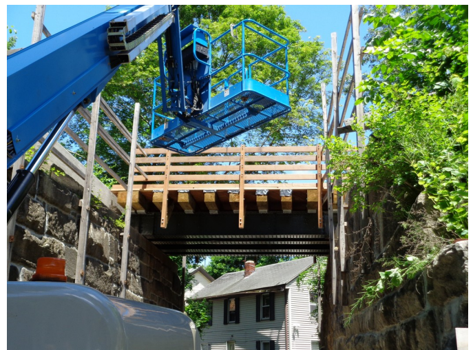
The Kane Court Bridge on 6/15/14
