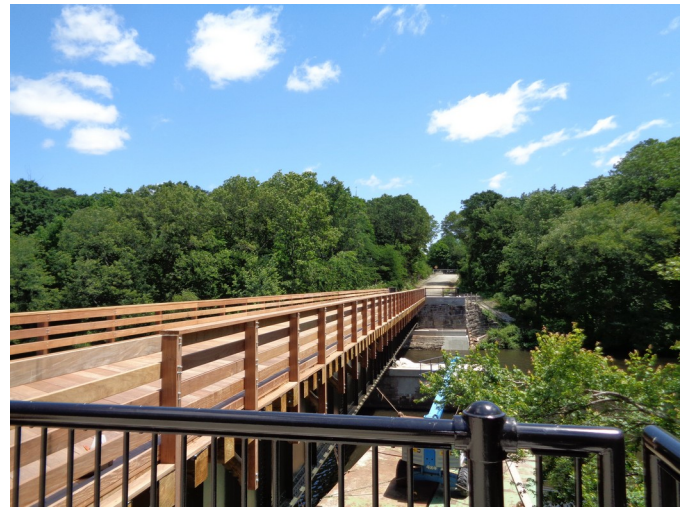
The longer Factory Pond Bridge looking east on 6/15/14
