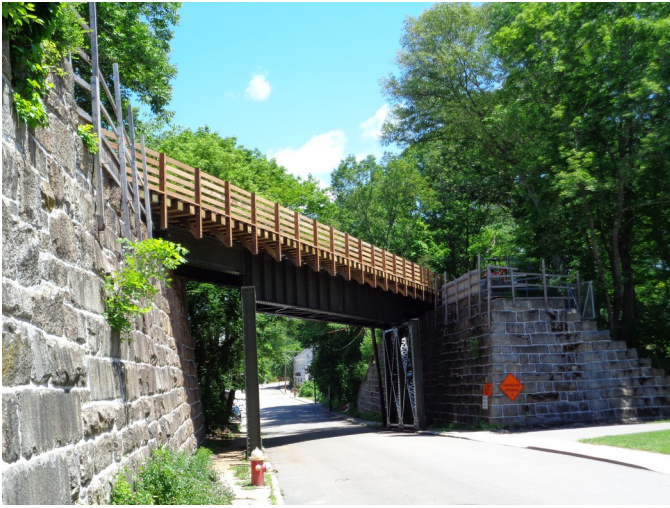
The Canal Street Bridge on 6/15/14 with deck & railings
