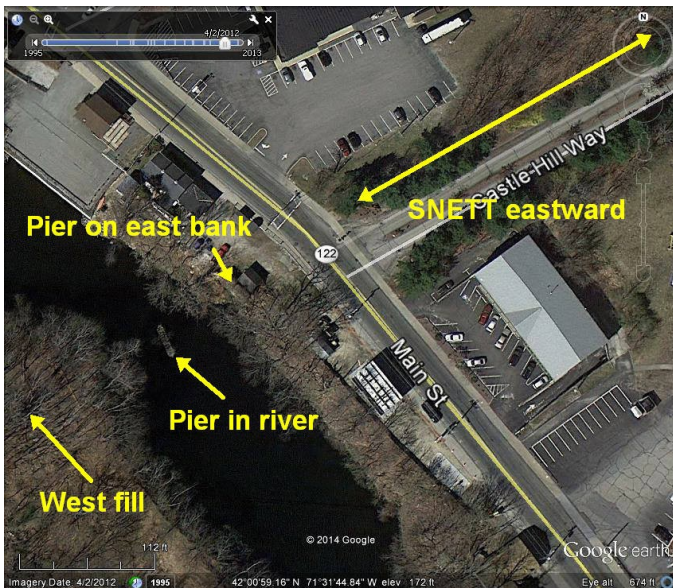
Aerial view of former railroad bridge site at Rte. 122 and Castle Hill Way, Blackstone
