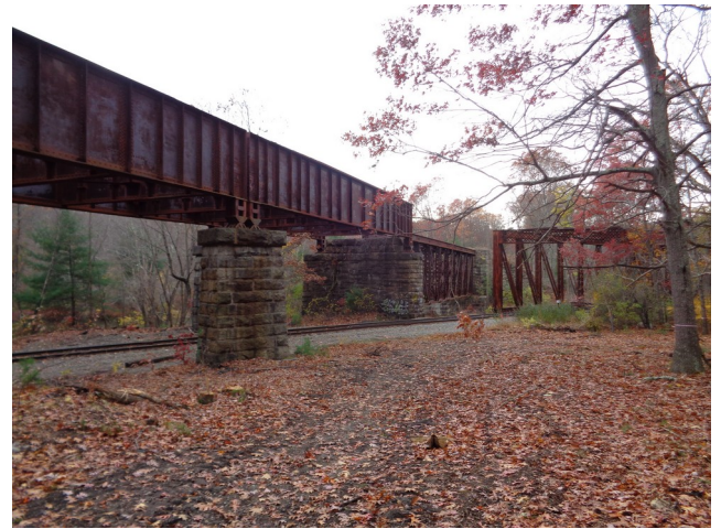
Triad SNETT bridge looking west on 11/2/14
