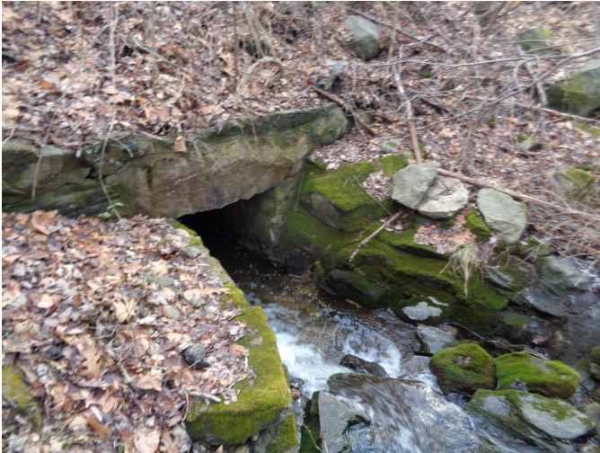
A culvert under the SNETT west of Fox Run Road, Bellingham
