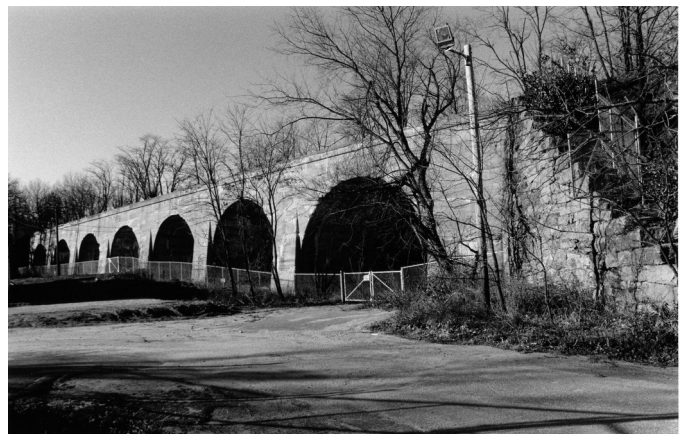
The seven arch section of the Blackstone Viaduct from the studies.
