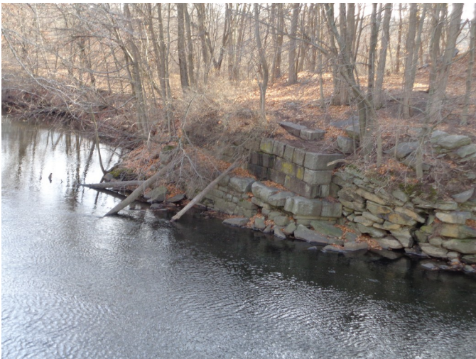
The remainder of the west abutment of the original bridge.
