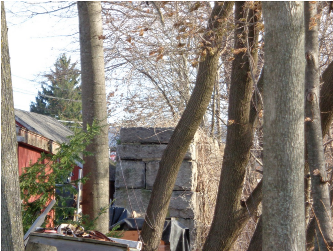
The north side of the intact east bank pier.
