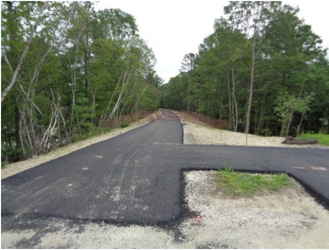
View looking eastward on the now paved SNETT at the top of the ramp at Adams Street, Uxbridge on 7/18/15. The pavement is not yet open for public use, but now extends to Central St. in Millville, MA.
