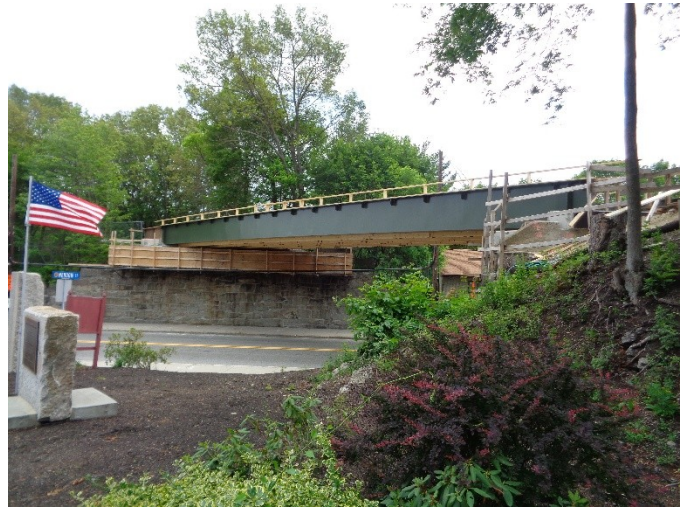
East face of the Main St. bridge 6/20/15
