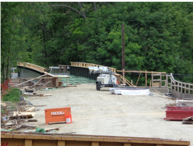
Looking south over the new Main St. bridge, Blackstone 6/20/15
