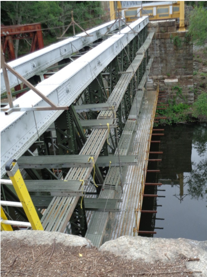
The layers of scaffolding on the SNETT Triad Bridge on 7/18/15.
