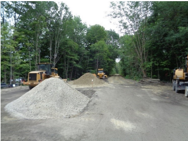
View on 7/18/15 looking eastward at Central St., Millville showing base work.
