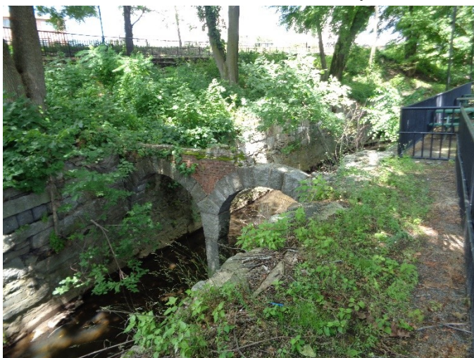
Arches on the power canals in Valley Falls Park 7/10/15
