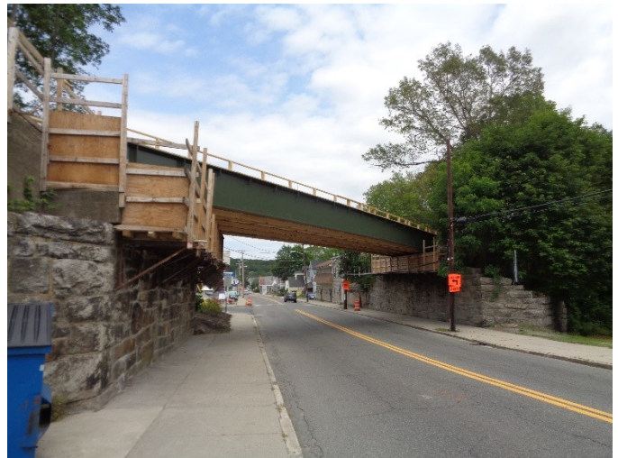
Eastward view of new Main St. Bridge, Blackstone. 6/20/15
