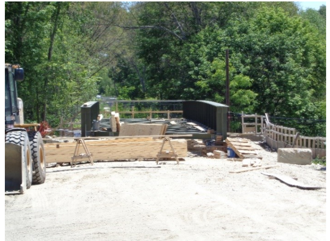
Main St. Bridge, Blackstone being assembled on 6/7/15
