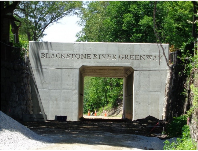
East face of Church St. Tunnel, Blackstone 6/7/15
