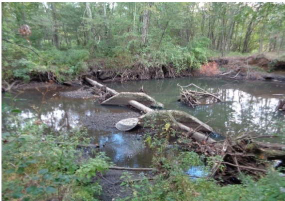
The old sewer line crossing on 9/19/15
