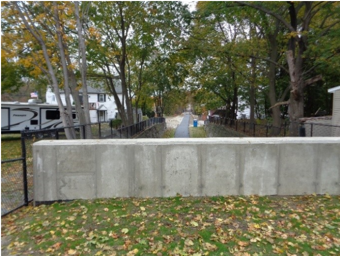
The view south of the Greenway from Church St., Blackstone towards Old Mendon St. and the depot, 10/28/15.
