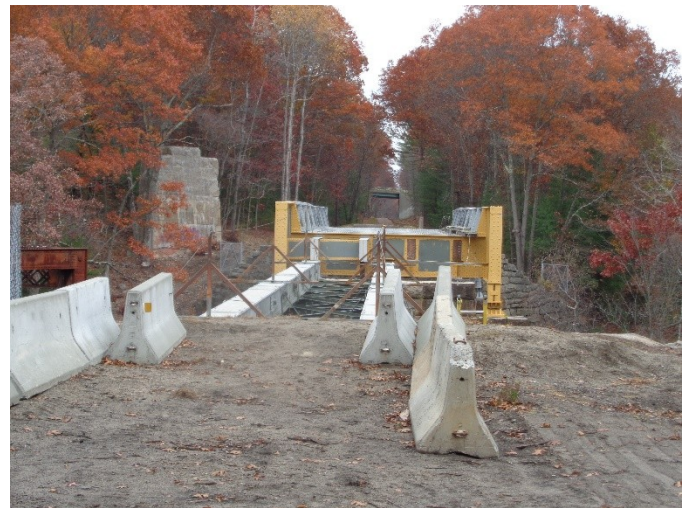
Triad Bridge looking east on 11/1/15. The "jersey" barriers are new.
