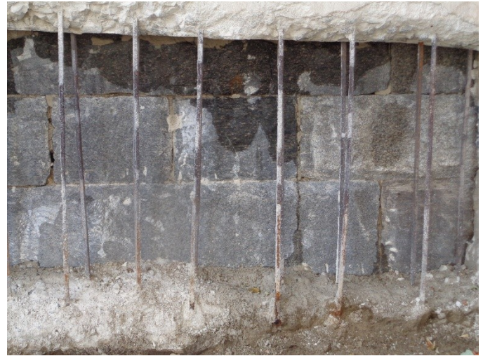
View of exposed masonry at lower part of eastern pier.
