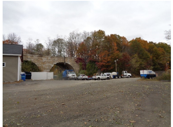
Blackstone Viaduct engineering testing work underway on 10/2/15
