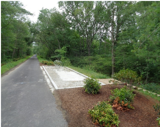
View looking westward along bikeway at side trail to Millville Lock on 7/10/16. Note the stairs on the right and the hoop bike racks. Pavers will probably be installed within the curbing.
