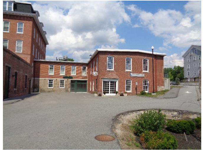
The new Corridor offices at the Linwood Mill, Northbridge, MA
