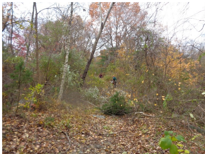
Trail clearance work underway on 11/5/16 looking west.
