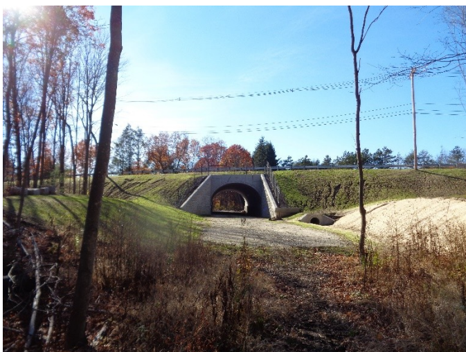
Looking westward along the SNETT towards the new Route 126 Tunnel on 11/7/16.
