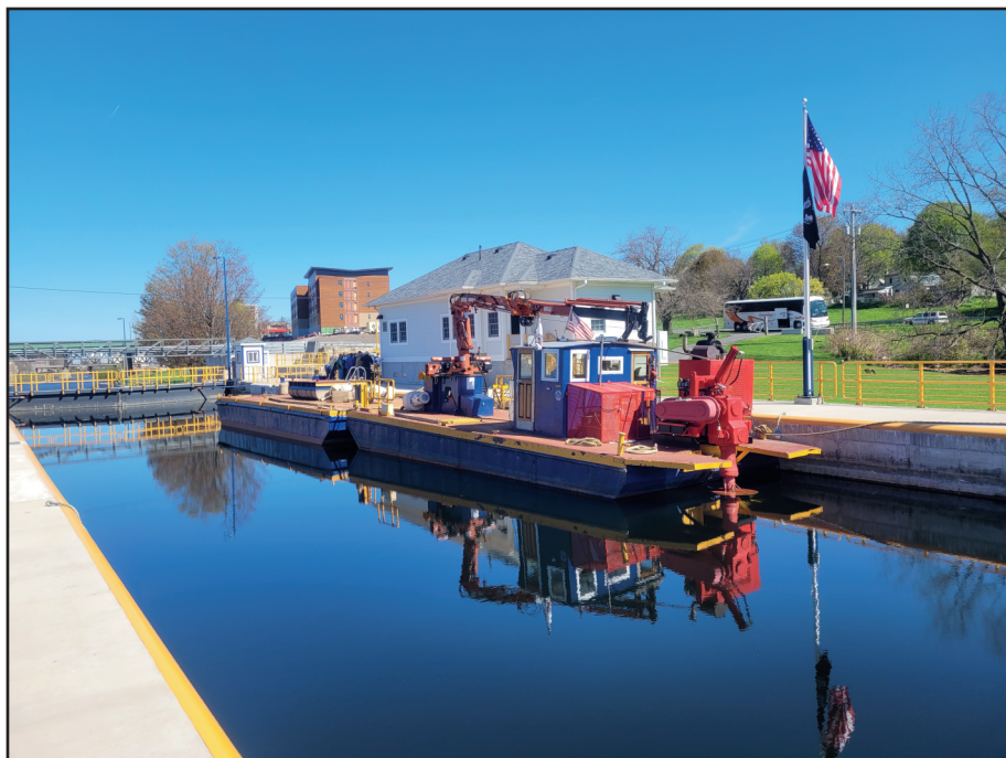
A workboat lies in the newly refurbished Oswego Canal Lock 7.
