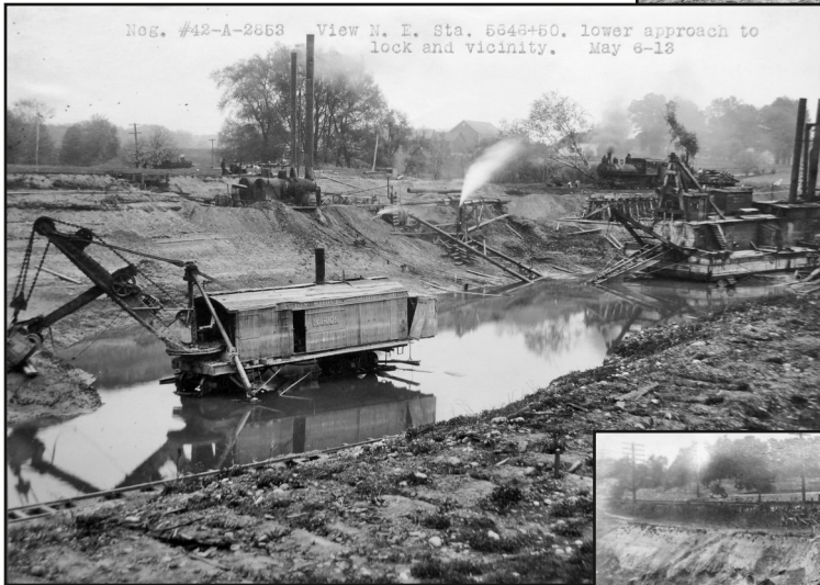
Above left – A variety of machines can be seen here on Contract 42-A. A Marion Model 60 sits cold in the pool of water while the dredge Mohawk sits just behind on the dry, while a steam pump works to drain the water.
