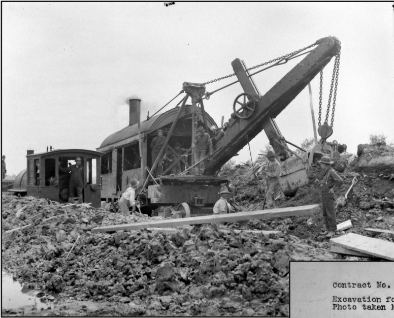
Facing Page and Top Left – This is likely the same shovel as seen on Contract 1. It appears to be a Marion model Improved -A, an older shovel at the time.
