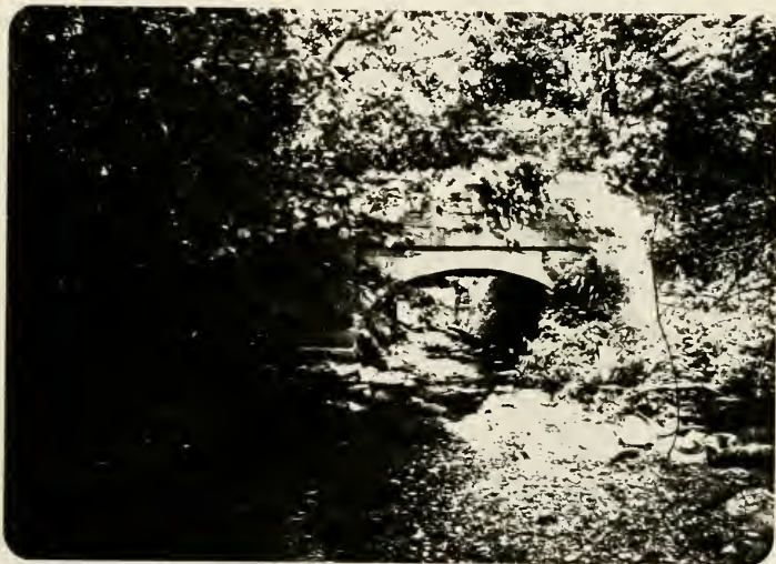
Plate 28. Haw's Double Culvert viewed from the south.
