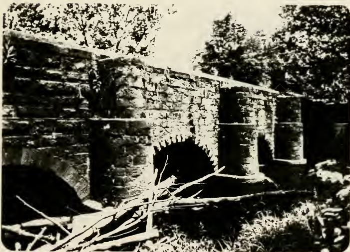
Plate 23. Unmatched and recycled stonework in the south wall of the Allegheny Aqueduct.
