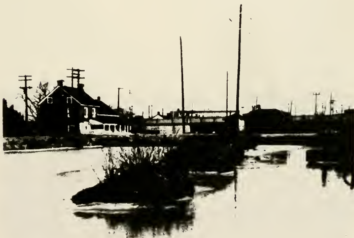
Plate 35. 1959 photograph taken from the lie-by above Lock No. 51; note the lockkeeper's residence on the left and the toll house on the right.
