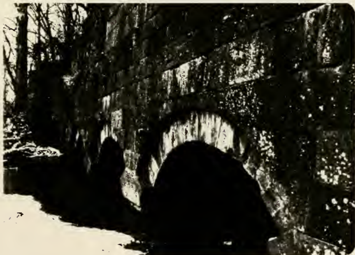
Plate 69. Detail of the arches in the north wall of Snyder's Culvert.
