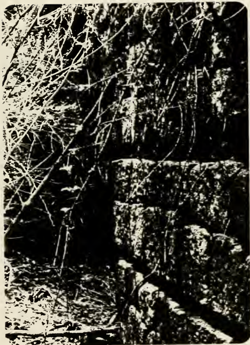
Plate 79. Miter gate pocket in the third chamber of the early triple locks at Laurel Hill.
