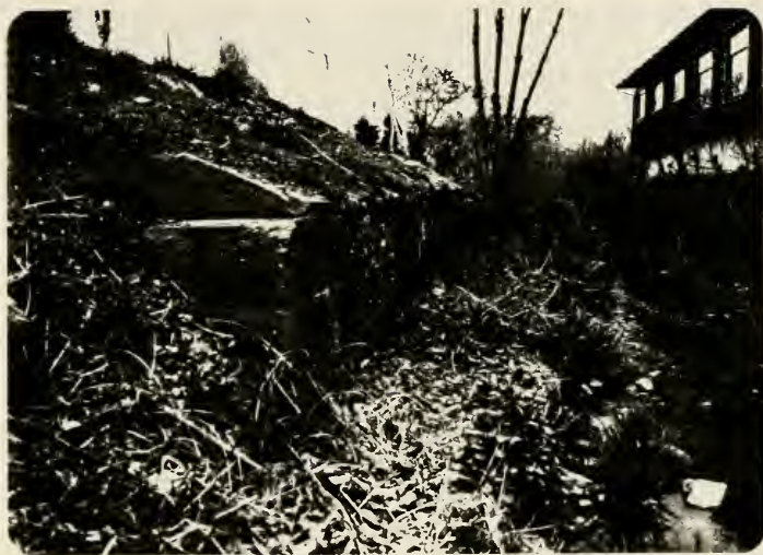
Plate 85. Ruin of Jones' Culvert.
