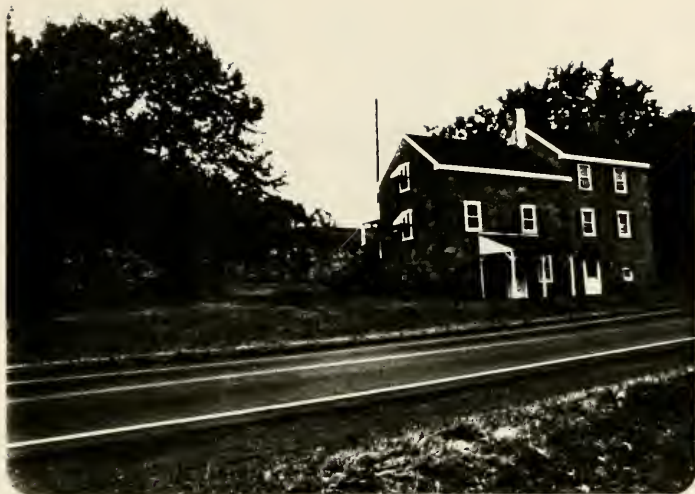
Plate 43. Lockkeeper's residence at Lock 51, Birdsboro Lock.
