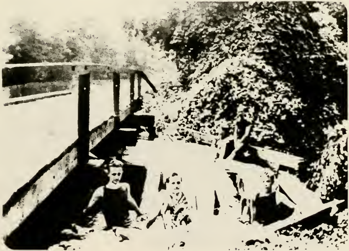
Plate 65. 1912 photograph showing children playing in the waste weir at Kirlin's Aqueduct; the tow path and canal are on the left edge of the photo.
