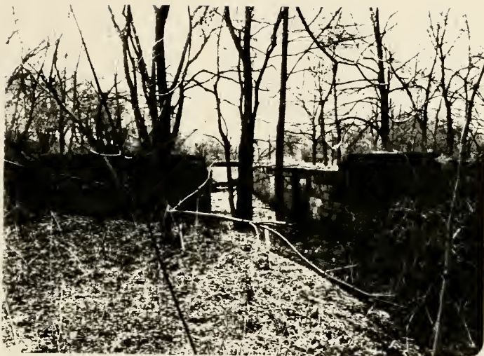
Plate 105. View of the Girard Outlet from the east. Note the tow path bridge abutments at the corners of the lock walls.
