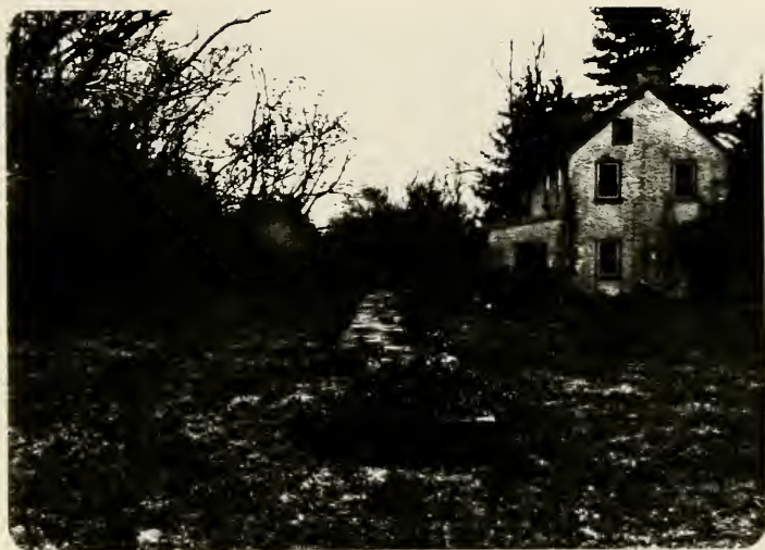
Plate 91. Filled upper chamber of Frick's Locks and the lockkeeper's residence.
