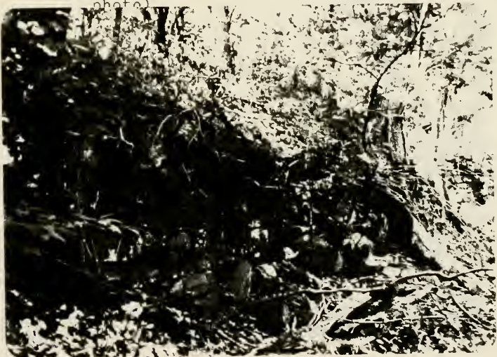
Plate 59. Retaining wall built on the north side of the tow path at the Monocacy Furnace Basin near Sixpenny Creek.
