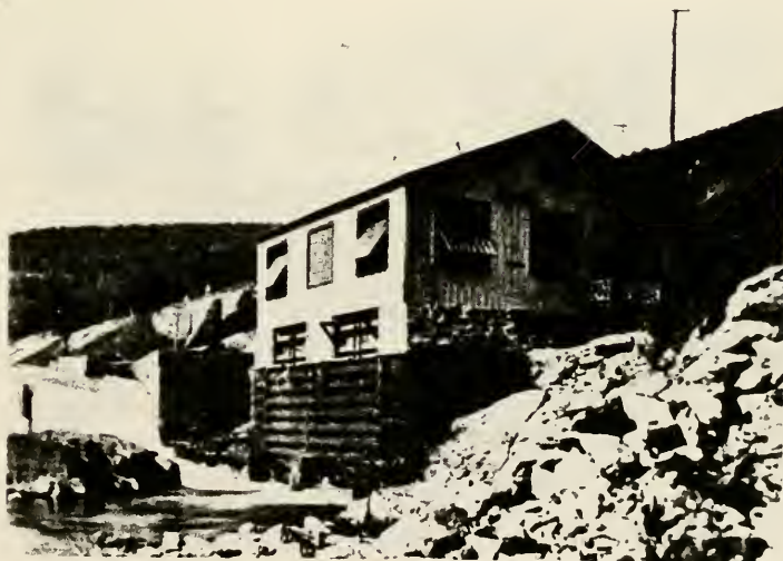
Plate 4. Southeast view of the Power House.
