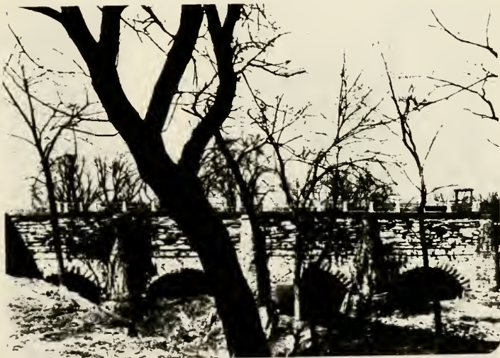
Plate 48. South wall of the Hay Creek Aqueduct photographed c. 1955.
