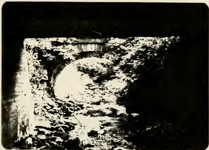
Plate 31. Modern bridge span resting on the old abutments of Haw's Road Bridge; in the background is the north side of the eastern arch of Haw's Double Culvert.
