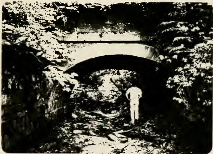
Plate 30. Western span of Haw's Double Culvert viewed from the north side.
