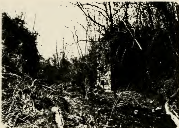
Plate 95. Ruin of Frick's Aqueduct viewed from the north.
