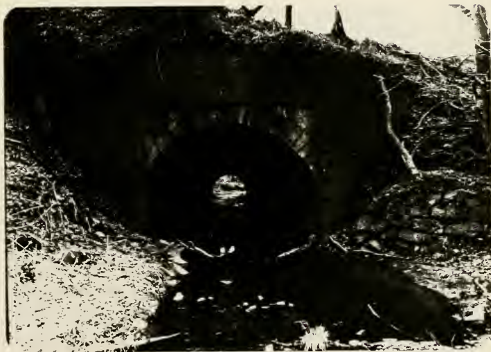
Plate 86. Grubb's Culvert viewed from the north.
