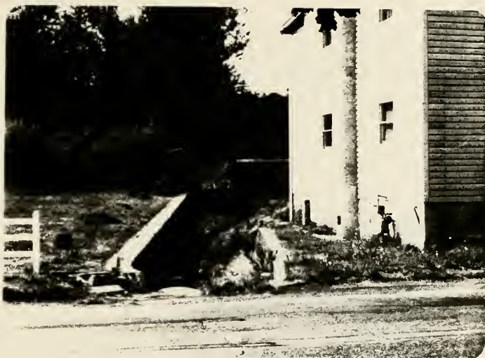
Plate 53. Ruins of the sluice built at Bland's Turn Waste Weir.
