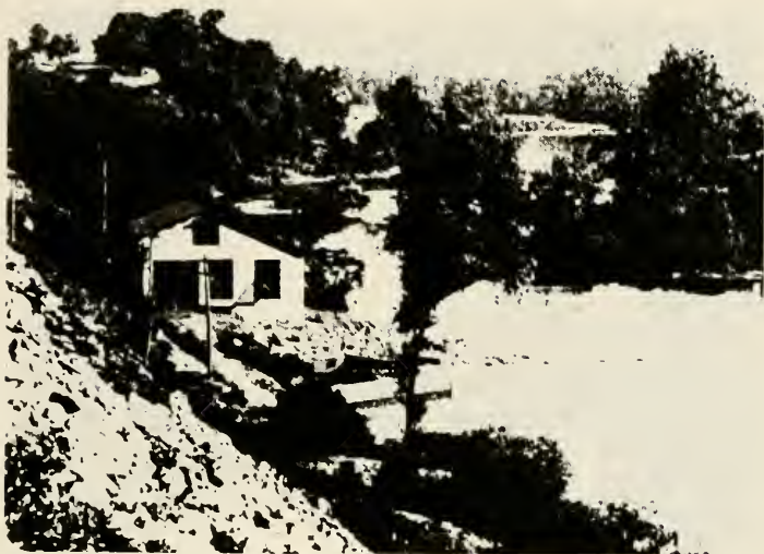
Plate 3. Power House at Dam No. 24 as seen from the north.
