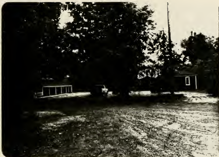
Plate 36. 1989 photograph taken from the filled lie-by above Lock No. 51; note the good condition of the buildings; the car is parked in the filled lock.
