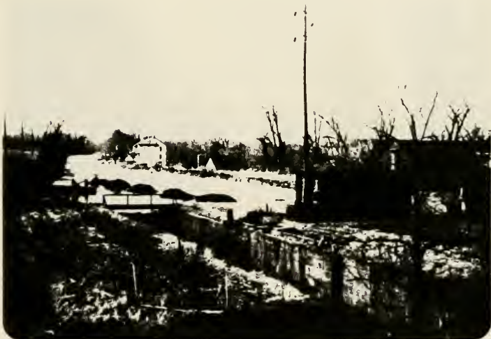
Plate 37. 1959 photograph showing the 1836 lock before it was filled.
