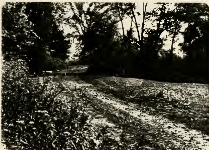
Plate 51. Site of Campbell's Road Bridge.
