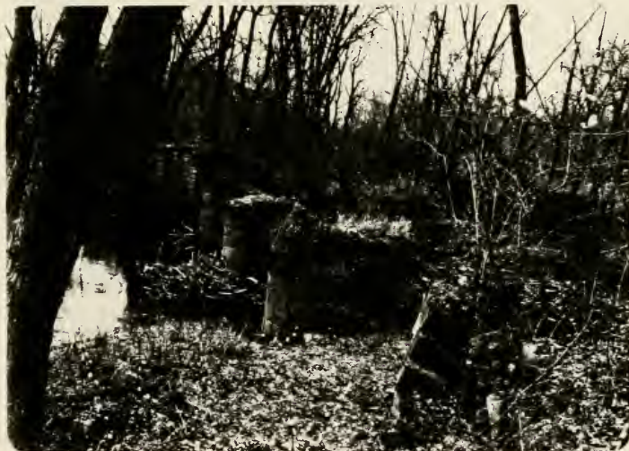
Plate 98. Ruin of Pigeon Creek Aqueduct.
