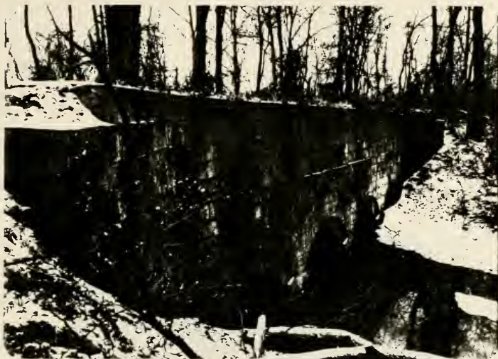
Plate 68. North side of Snyder's Culvert.
