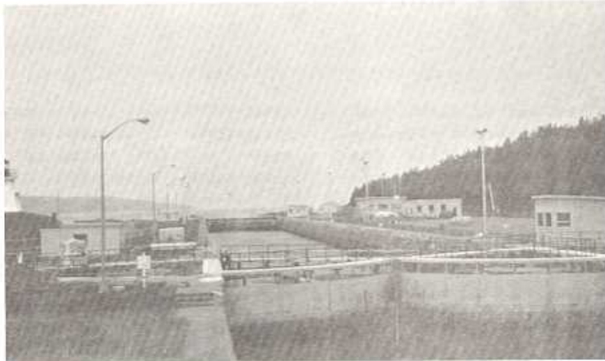
THE CANSO CANAL AND SINGLE LOCK, 1987. PHOTOGRAPH TAKEN FROM THE COMBINED ROAD AND RAIL SWING BRIDGE AT THE SOUTH EAST END. Photo By Colin Duquemin
