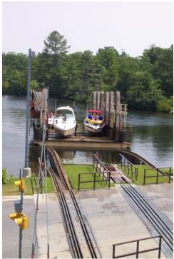
There is a second alternative and that is to use a Marine Railway, such as the one at Big Chute on the Trent-Severn Waterway. This could raise boats high enough to provide the railway with the clearance that it needs. A Marine Railway could be a tourist attraction in its own right.
