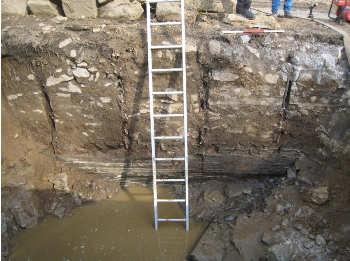
Photograph 3 - Inside face of the north lock wall. There are recesses in the wall for embedded timbers and the remains of horizontal wood planking near the bottom of the wall.
