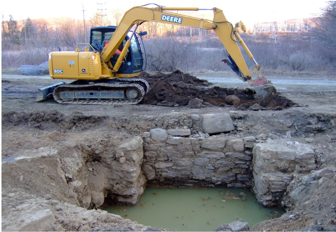
Photograph 2 - The outside face of the south lock wall has stone buttresses that protrude from the face of the wall. These allow a thinner wall between the buttresses.
