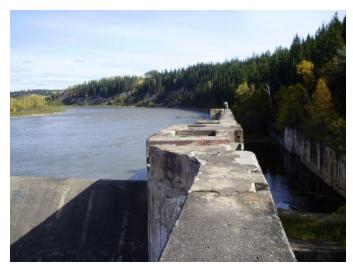
An engineer from the Niagara region, Charles Mitchell, proposed to build a 3.8 m overflow dam in the river. Although time was of the essence, the following vear engineering consultants from Toronto recommended major changes to the original plan, including a 7 m high dam. With the revised plans - and price approved bv City Council. construction started in 1912. In the summer of 1913 though, with 1/3 of the dam finished, more
