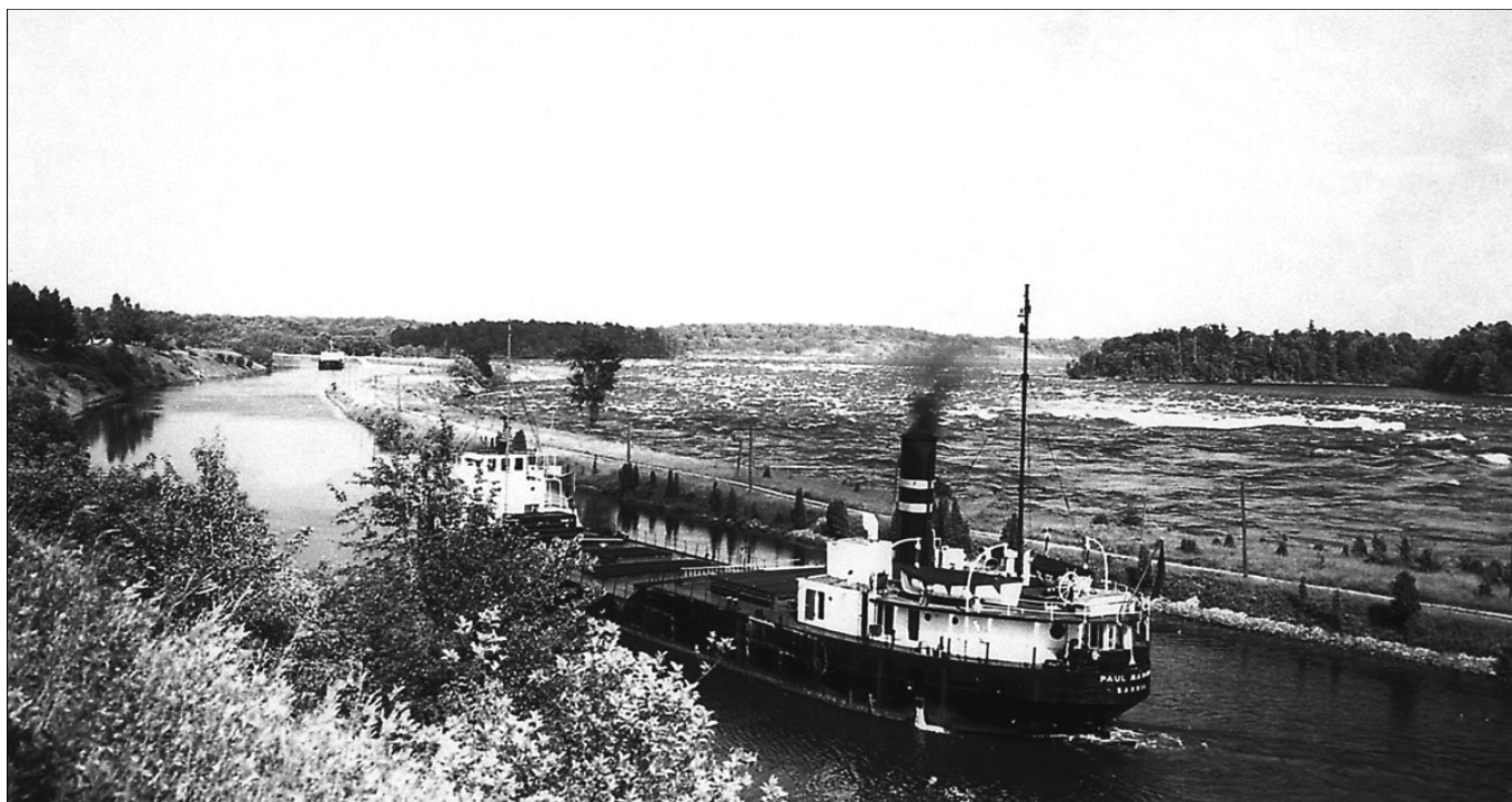
A view of the Cornwall Canal, showing the fast water of the Long Sault Rapids in the background.
