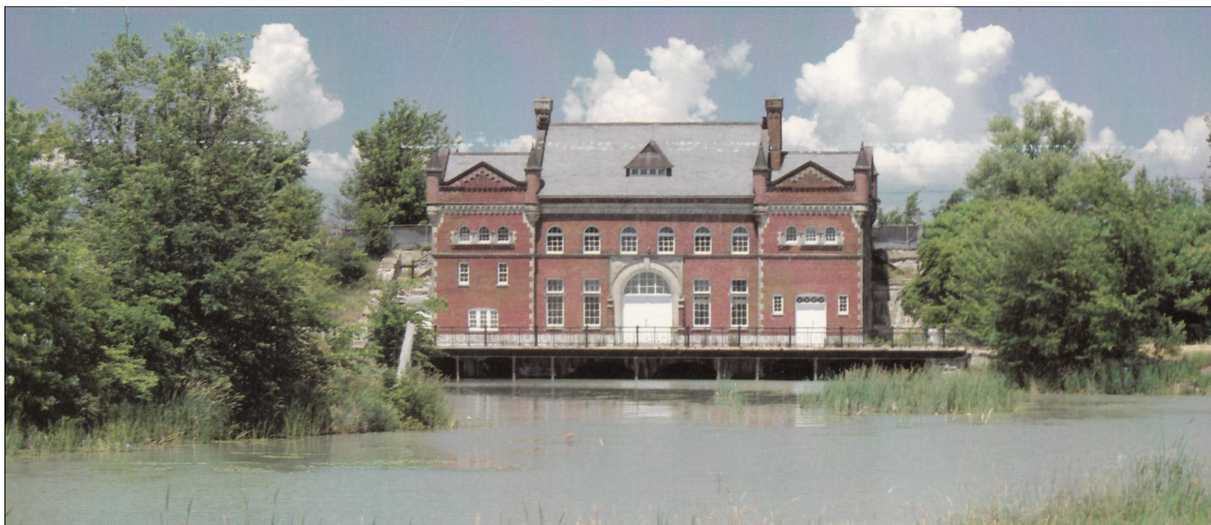
The Le Petit Pouvoir , the small power house built to provide electricity along the Soulanges Canal. This building still stands and can be seen from both the Chemin du Canal and the Chemin du Fleuve.
